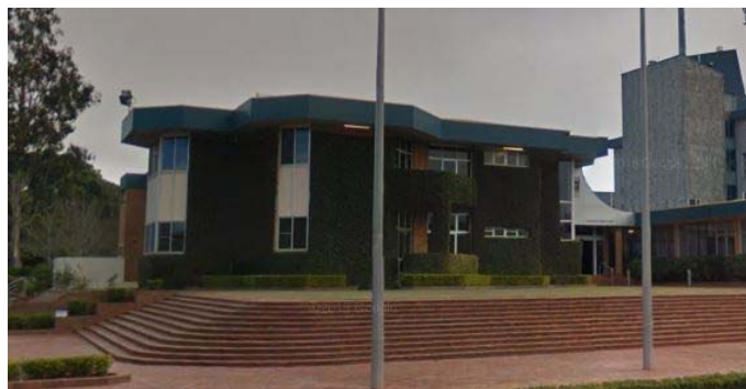
Figure 3.3: Parts of wall covered in vegetation
