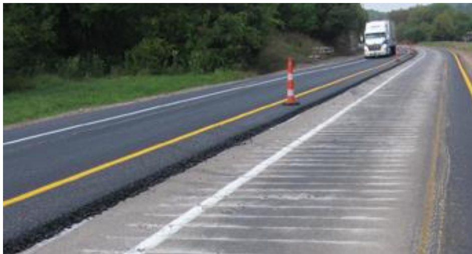
Figure 3: Asphalt overlay, Kentucky USA
