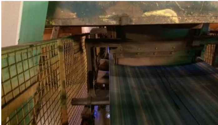
Figure B-4 Flattening of belt at chute outlet.
