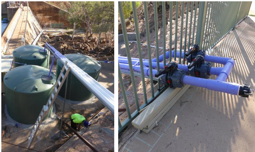
Figure 4.5 – Polyaluminium Chloride Installation Work in Progress (Molloy 2016)
