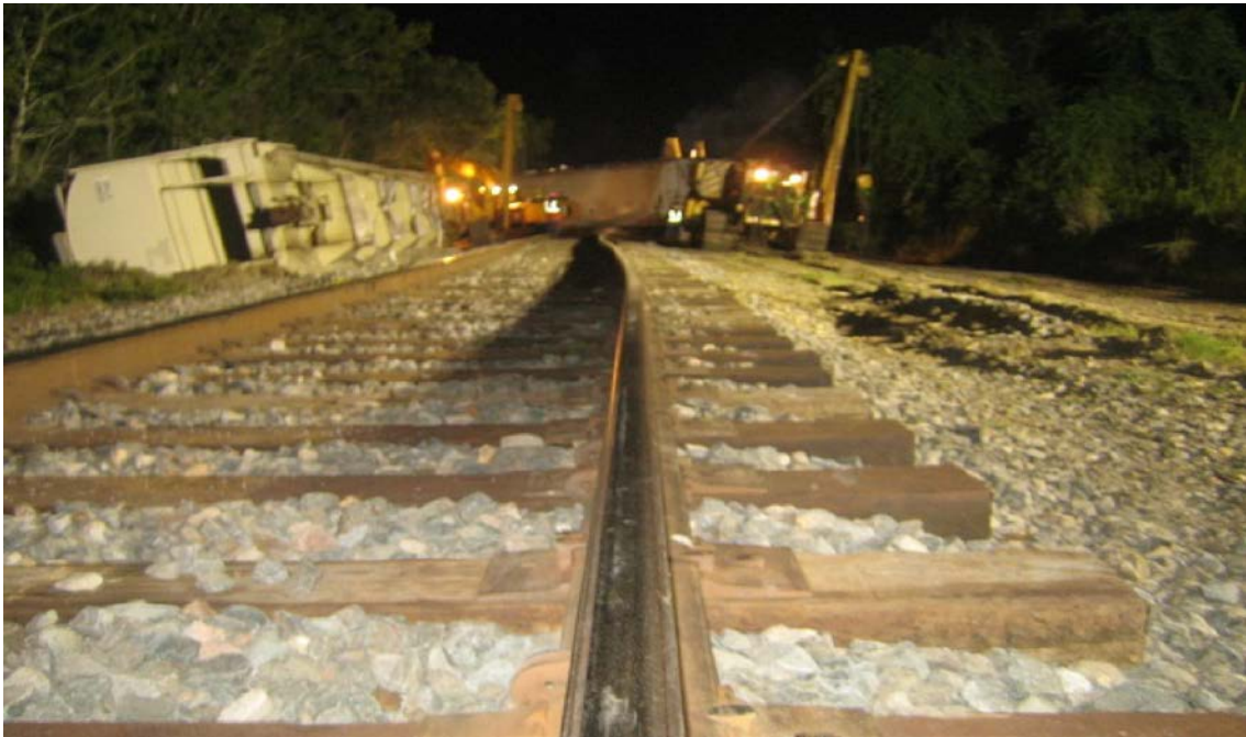
Figure 2-9: Derailment due to Track Buckling (Kish 2011)
