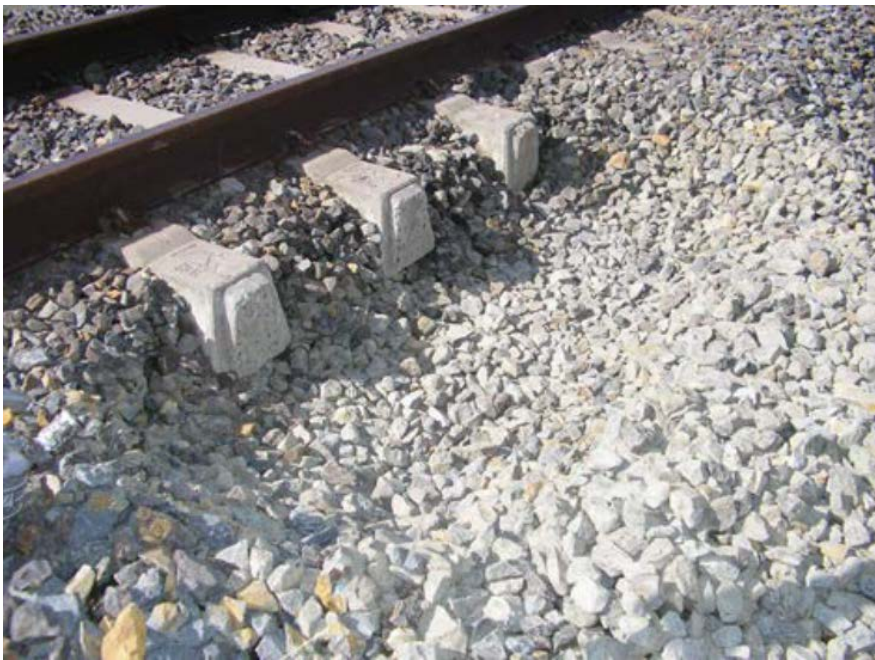
Figure 2-16: Excavation Required to Perform Test
