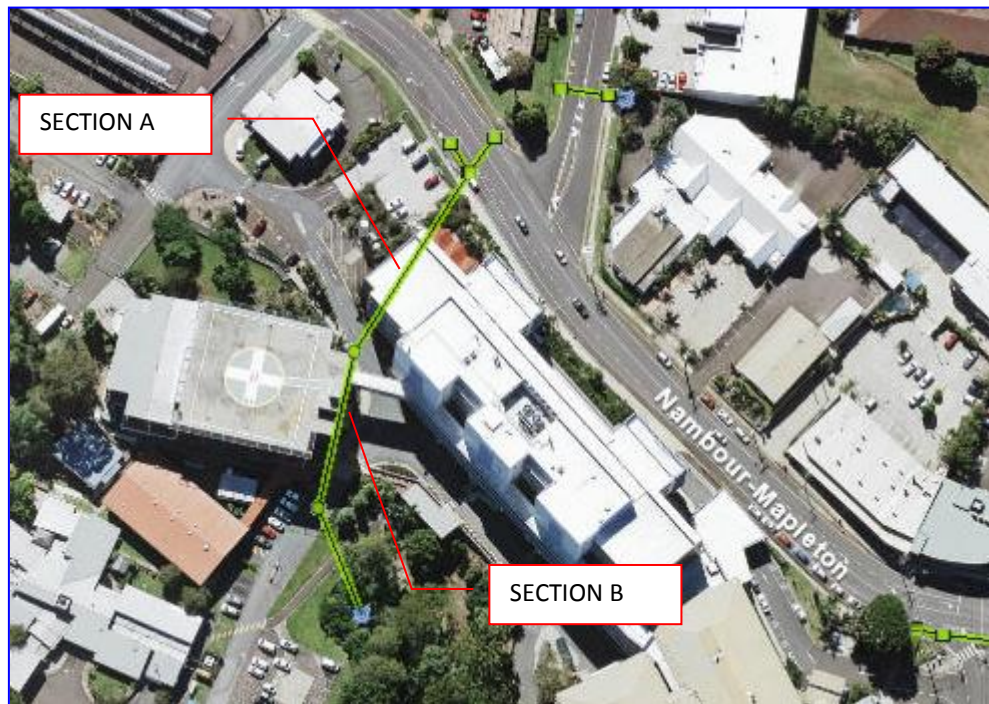
Figure 6.1: Sample Network A - Nambour Hospital (SCC GIS 2016)
