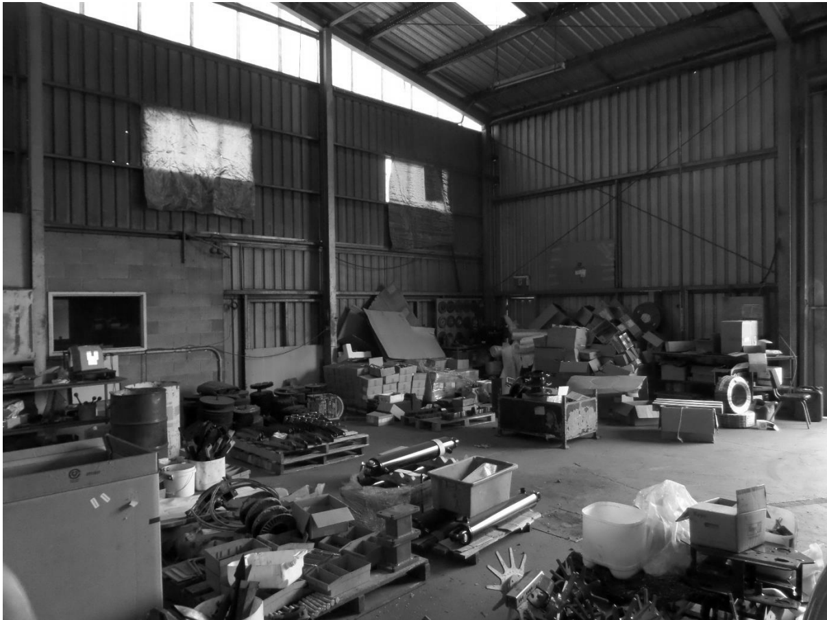
Figure 14 - The former stores area. This demonstrates the worst possible conditions
