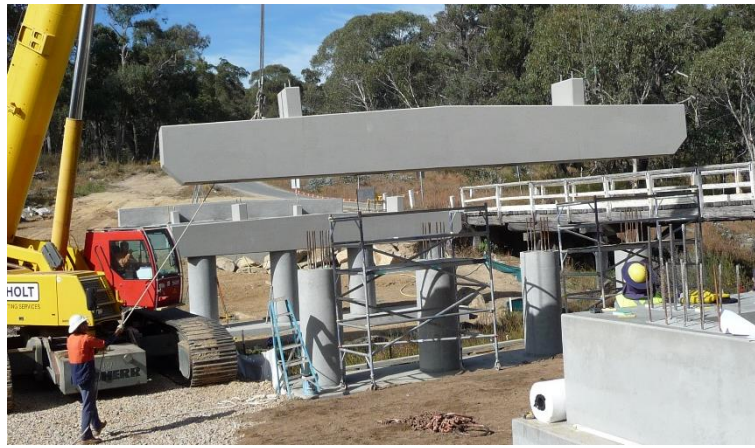
Figure 4-23 - Lowering a precast head stock
