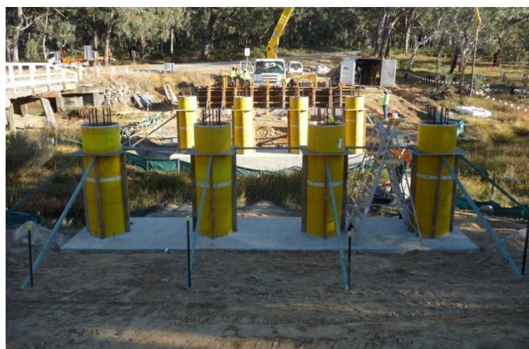
Figure 4-16 - Column formwork and falsework
