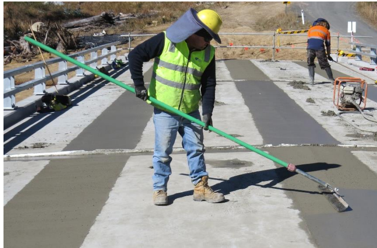
Figure 4-50 - Broom finishing deck concrete
