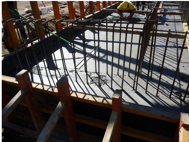
Figure 4-14 - Finishing concrete at Abutment B
