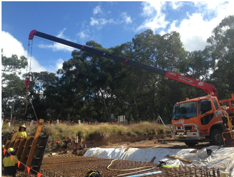
Figure 4-12 - Installing recycled formwork to Abutment B
