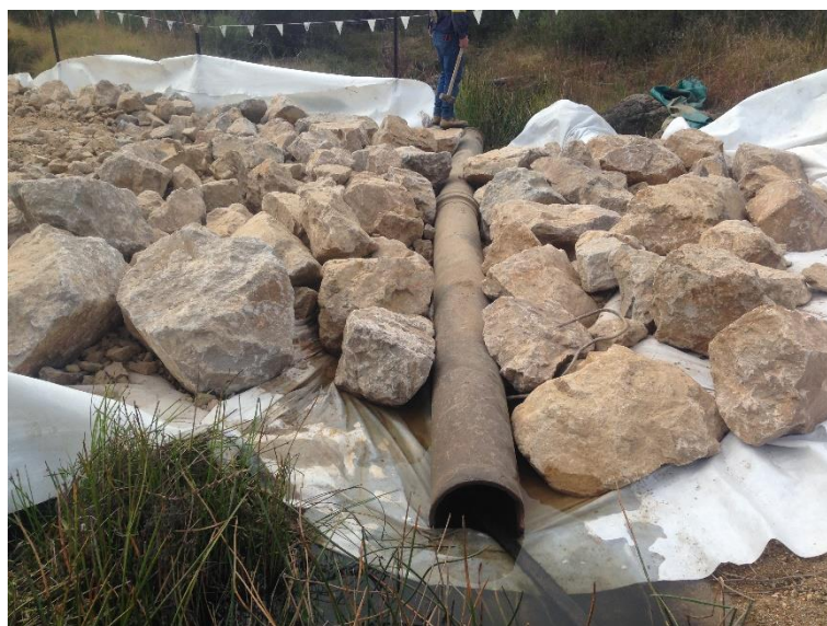
Figure 4-20 - Installation of creek crossing
