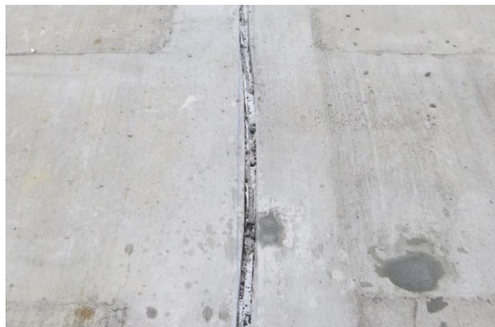
Figure 5-23 - Joint alignment issue
