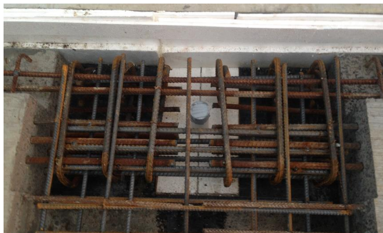
Figure 4-45 - Completed reinforcement in end diaphragm
