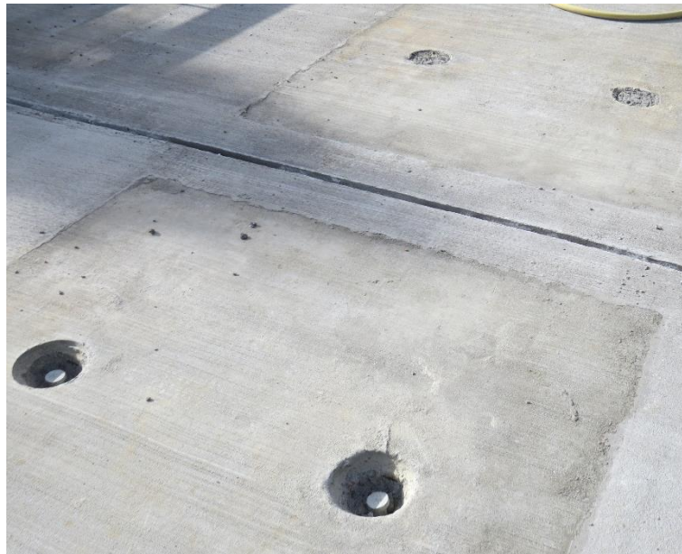
Figure 4-56 - Grouting of deck lifting points
