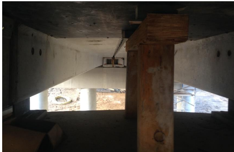
Figure 4-46 - End diaphragm soffit formwork
