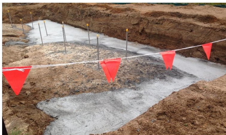
Figure 4-8 - Concrete blinding and dowels at Abutment B
