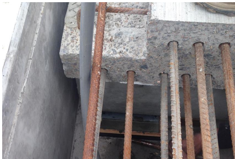
Figure 5-8 - End diaphragm projected reinforcement
