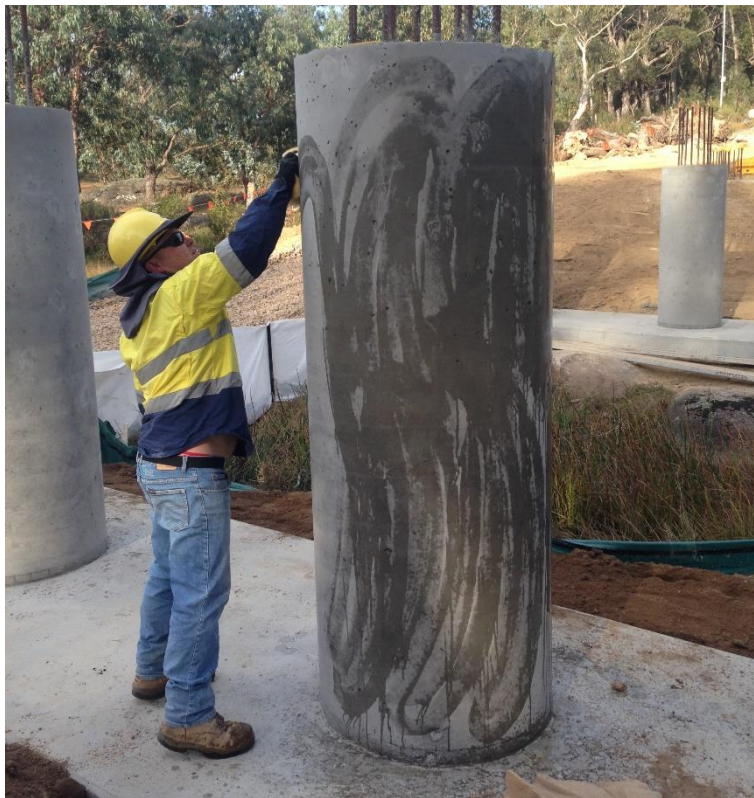
Figure 4-18 - Bagging Pier columns
