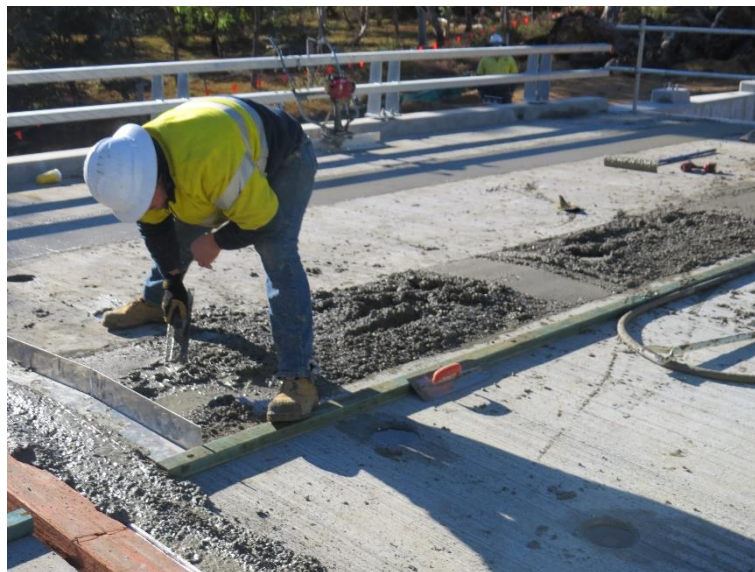
Figure 4-47 - Screeding deck central closure strip including cross fall apex
