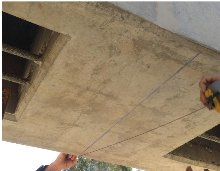
Figure 4-22 - Marking chalk lines on precast headstock
