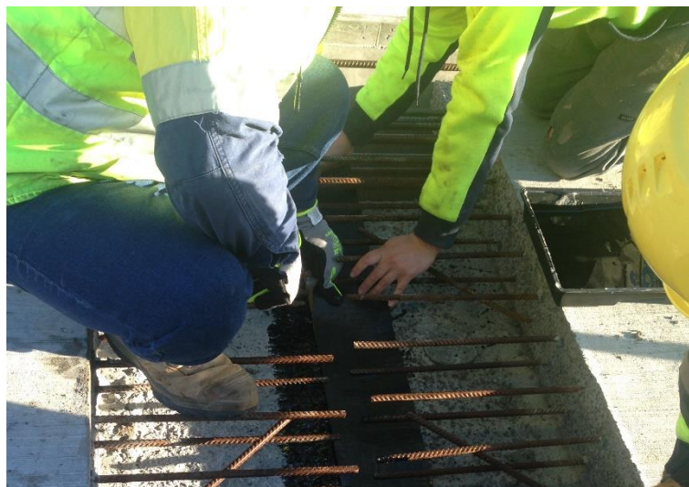
Figure 4-40 - Sealing gap between deck module flanges
