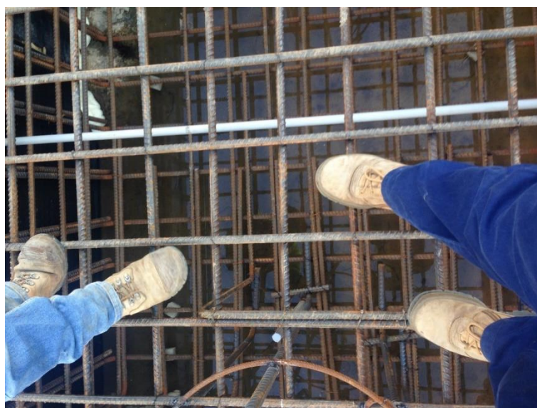
Figure 5-1 - Spacing of reinforcement
