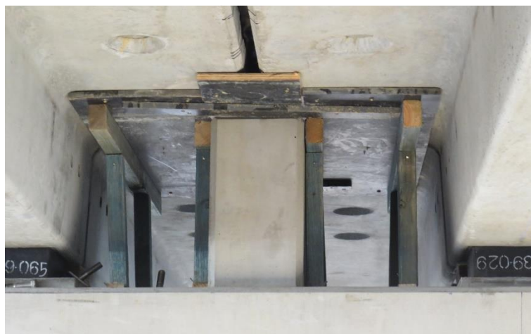
Figure 6-13 - Soffit formwork around shear key
