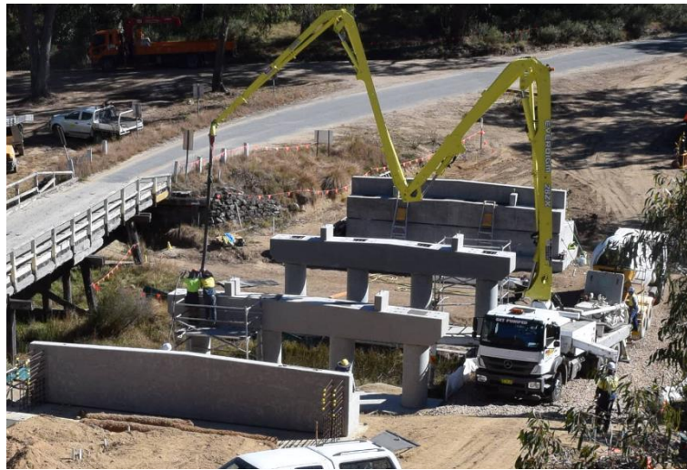
Figure 4-25 - Pouring concrete for column to head stock stitch
