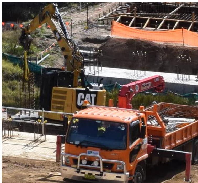
Figure 4-15 - Installation of column reinforcement cage
