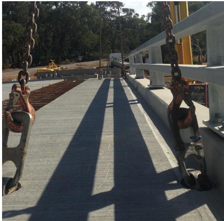
Figure 4-26 - Lifting arrangement for precast deck module
