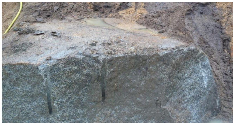
Figure 4-7 - Rock splitting in Pier One
