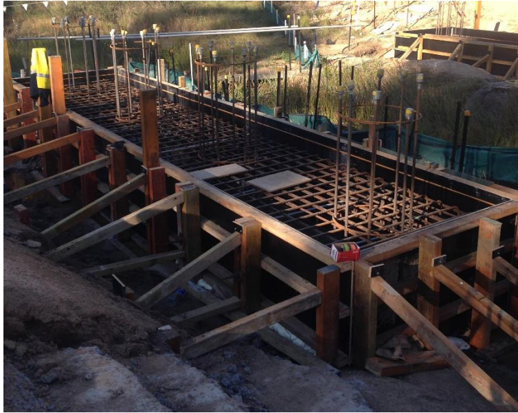
Figure 4-11 - Steel cage, formwork and falsework for Pier Two
