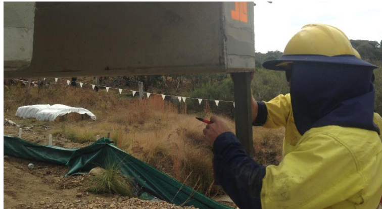
Figure 4-27 - Marking chalk line on precast deck module
