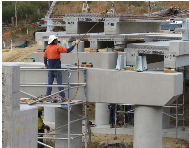
Figure 4-28 - Lowering an internal deck module
