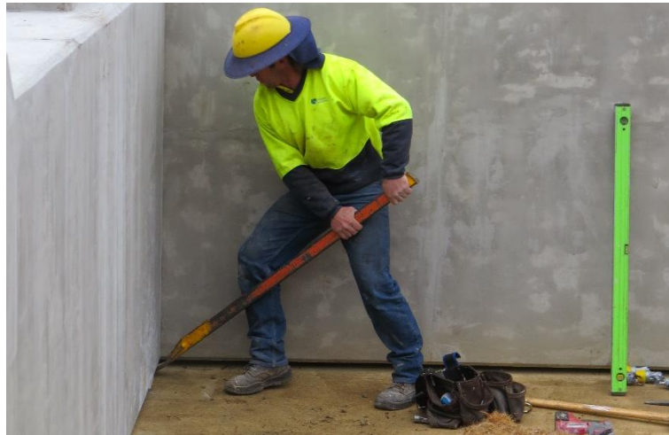
Figure 4-34 - Adjustment of precast wing wall position
