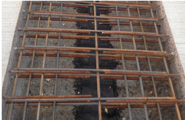
Figure 4-44 – Completed reinforcement above deck module flanges
