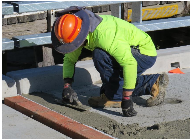
Figure 4-48 - Screeding transverse closure pour near expansion joint
