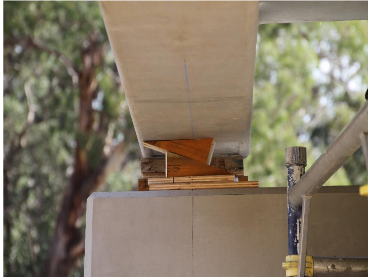
Figure 4-30 - Internal deck module installed
