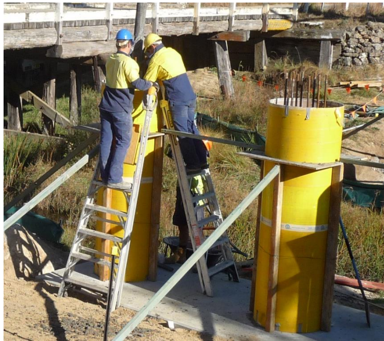
Figure 4-17 - Pouring concrete for Pier columns
