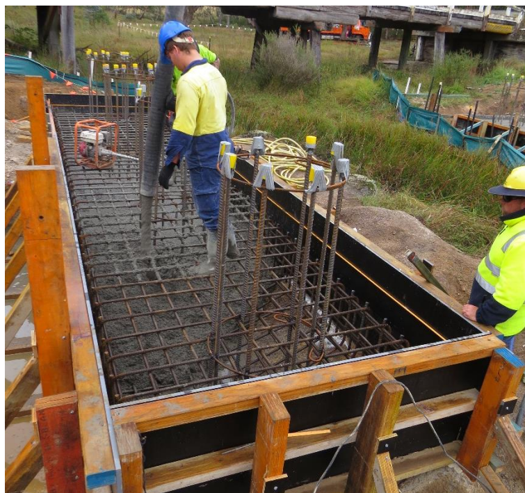
Figure 4-13 - Pouring concrete for Pier One footing
