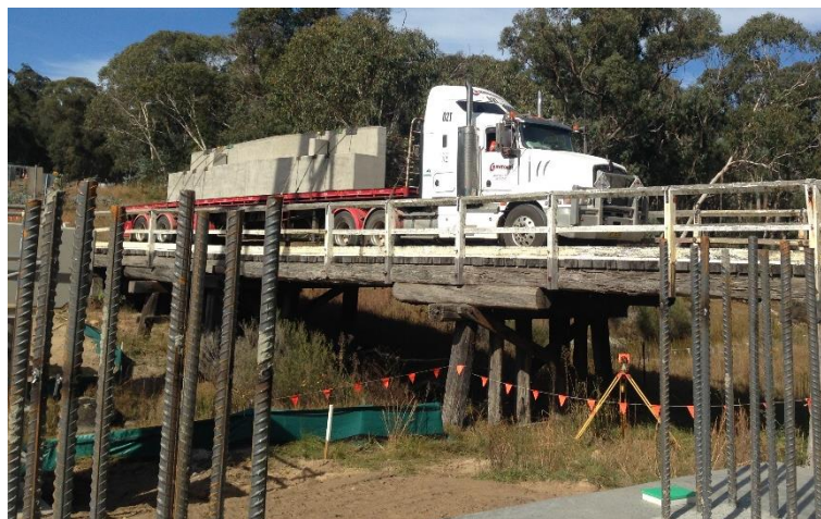
Figure 4-21 - Delivery of sill beam
