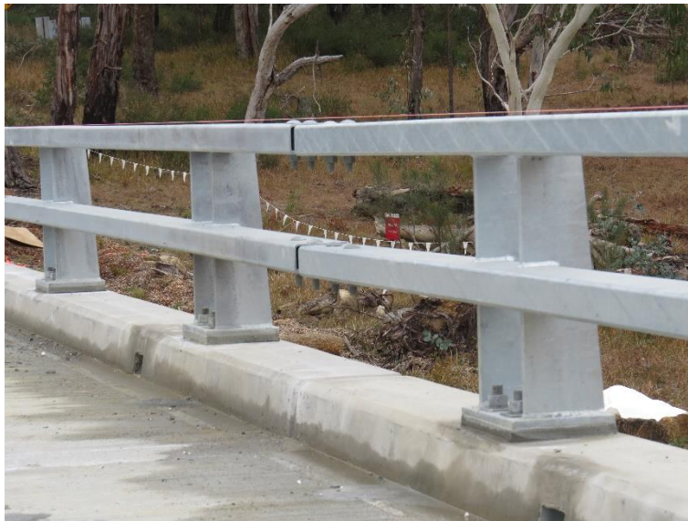
Figure 4-53 - Completed traffic barrier
