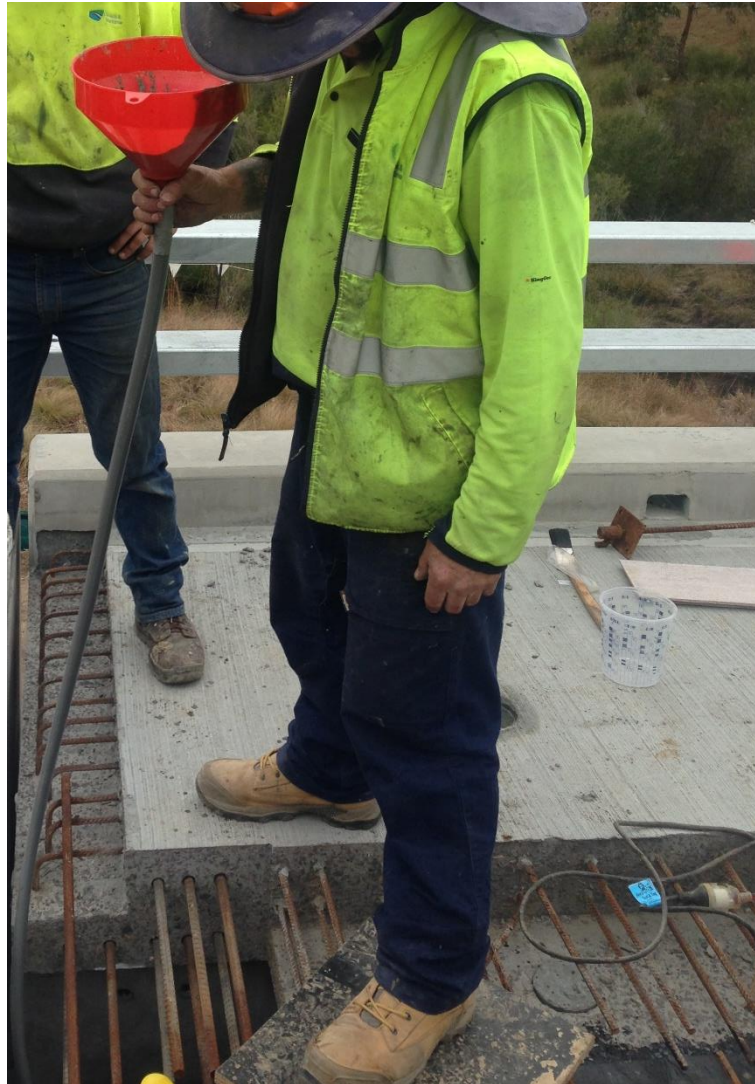
Figure 4-41 - Pouring grout to bearings
