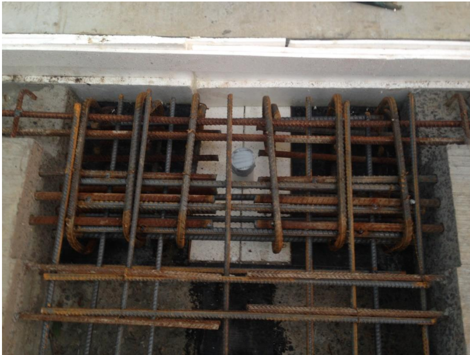
Figure 5-15 - End diaphragm reinforcement congestion
