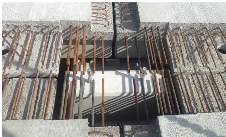
Figure 4-42 - Shear key at Pier One
