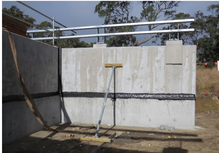
Figure 4-54 - Sealing the back of the Abutment
