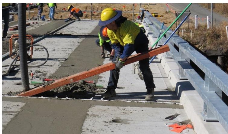
Figure 4-49 - Removing timber formwork brace from transverse joint
