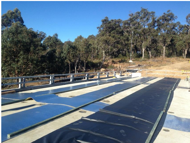
Figure 4-51 - Thermal protection of deck closure strip concrete
