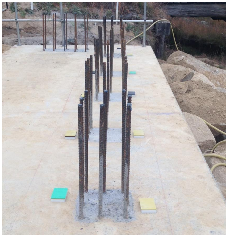
Figure 4-19 - Packers and chalk line marking at Abutment B footing
