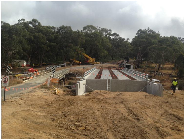
Figure 4-36 - Site after installation of deck modules and wing walls
