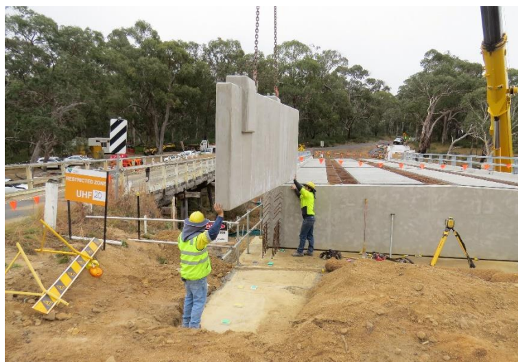
Figure 4-33 - Lowering precast wing wall into position
