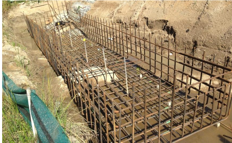
Figure 4-10 - Steel cage for Pier Two
