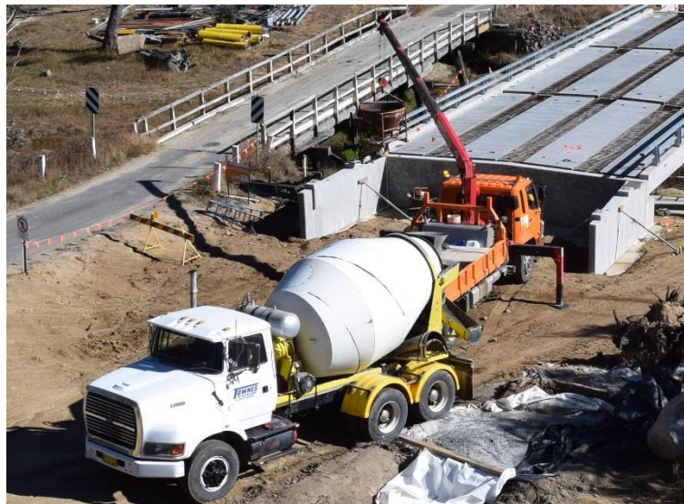
Figure 4-37 - Placing wing wall stitch concrete
