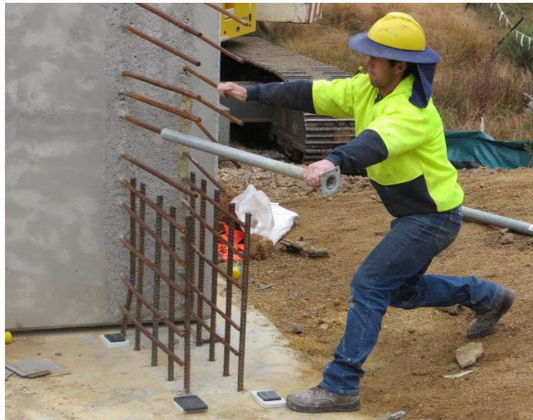
Figure 4-32 - Adjusting sill beam projected reinforcement
