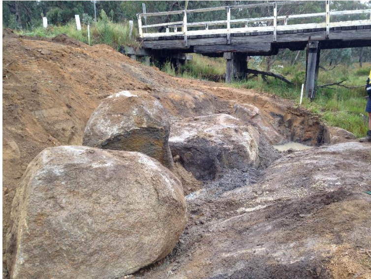
Figure 4-6 - Excavation of Pier One
