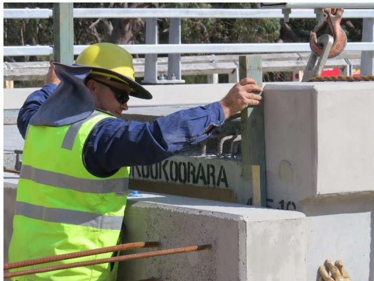
Figure 4-29 - Setting joint gap between deck module and Abutment
