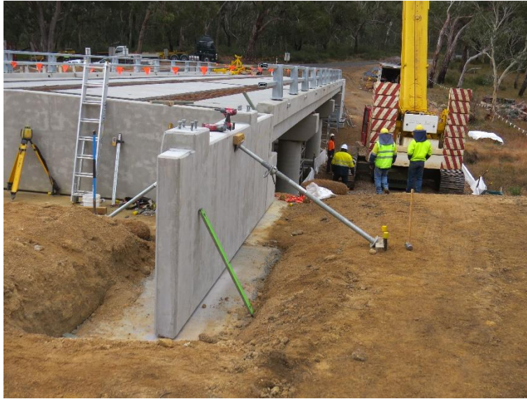
Figure 4-35 - Bracing of placed precast wing wall
