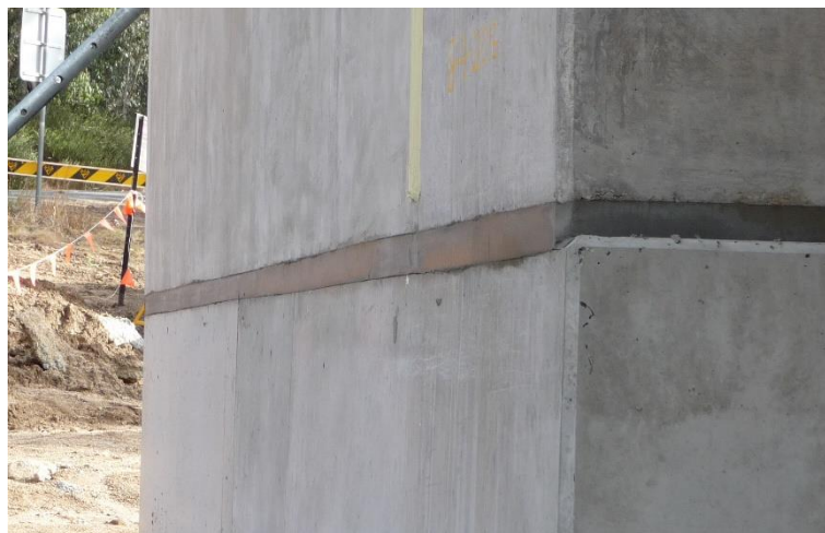
Figure 4-55 - Completed Abutment and wing wall face
