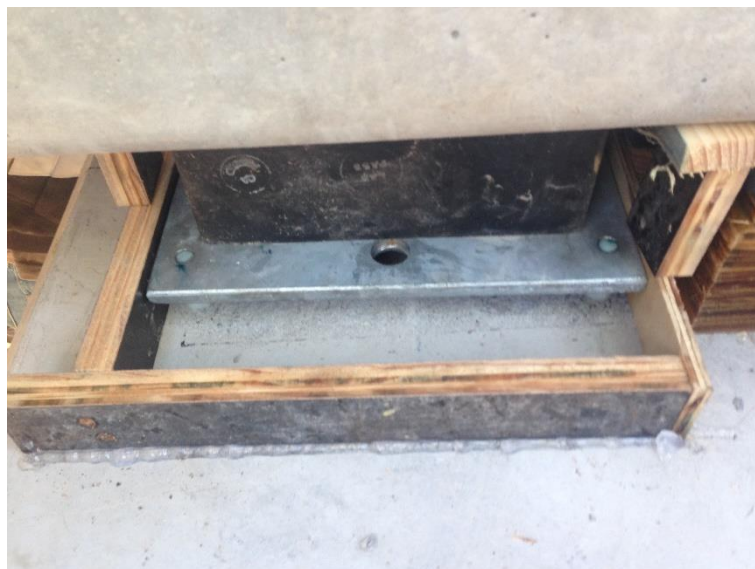
Figure 4-39 - Bearing formwork
