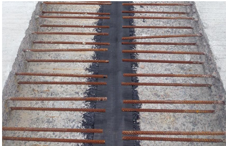
Figure 4-43 - Projected reinforcement above deck module flanges
