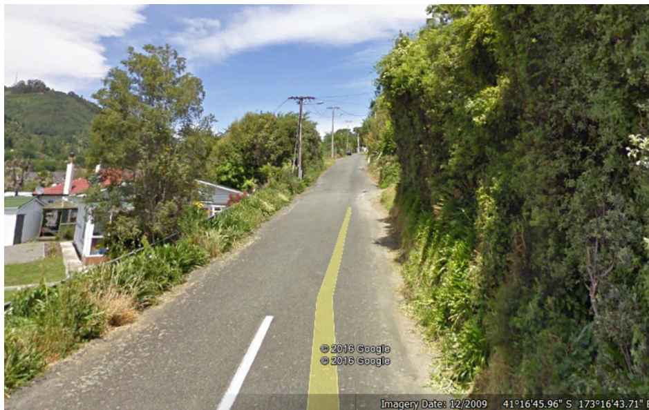
Figure 2.1 – Locking Street prior to road upgrade (Google Street View, 2016)
