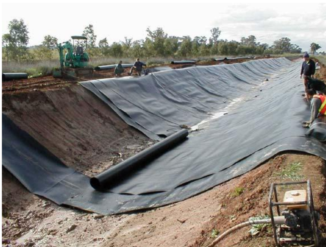
Figure 2.2: A channel being lined with a HDPE (ANCID 2004).
