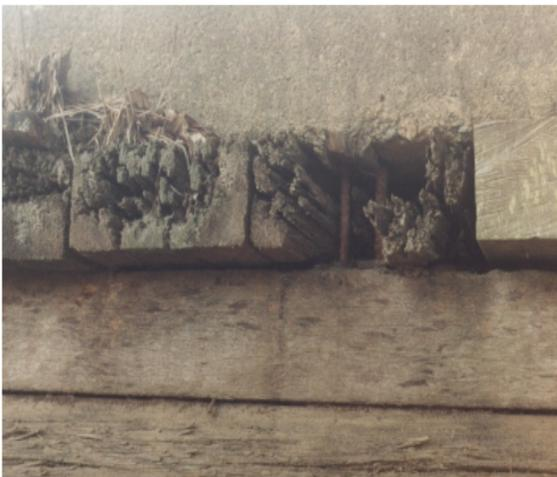
**Figure 2.5** - Rotted Ends of Deck Planks
