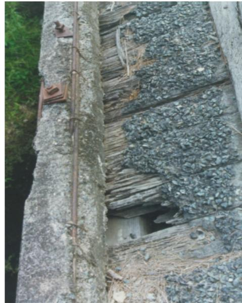
**Figure 2.6** - Weathered and Rotted Timber deck Planks
