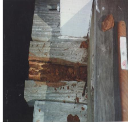
**Figure 2.2** - Termite Damage in Deck Planks
