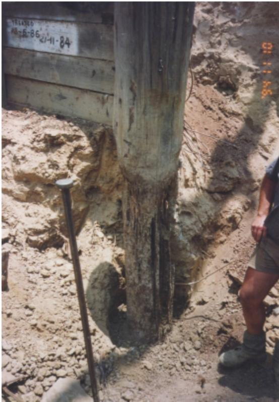
**Figure 2.7** – Rotting of Abutment pile below ground level (possible marine deterioration)
