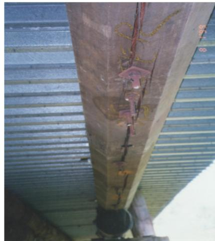
**Figure 2.4** - Splitting in Girder
