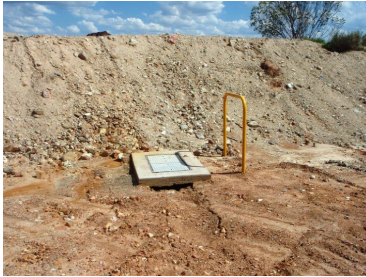
Figure 77 – Erosion and cracking around WE3 installation
