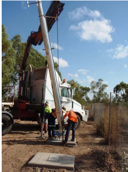
Figure 58 – Lifting hinged pole into place with truck mounted crane
