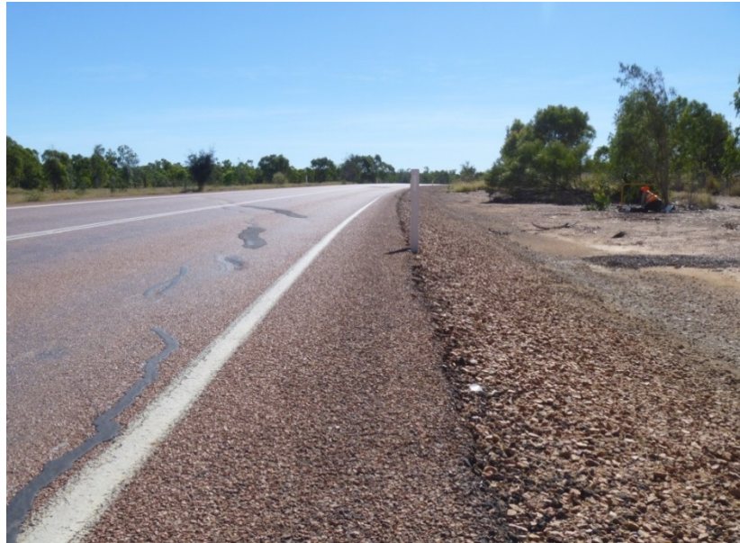
Figure 38 – Repaired pavement cracking, July 2013
