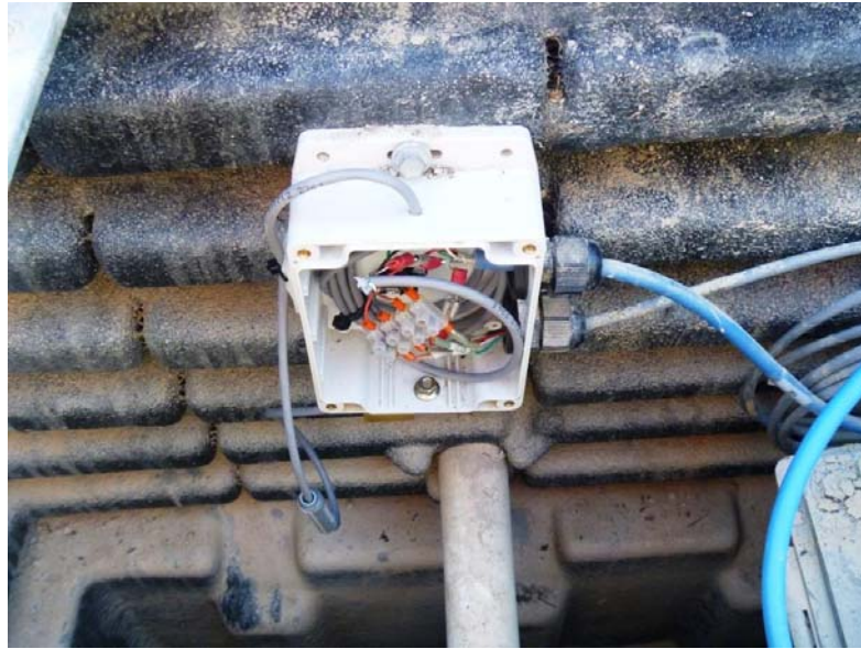
Figure 62 – Temperature sensor bolted to bottom of junction box
