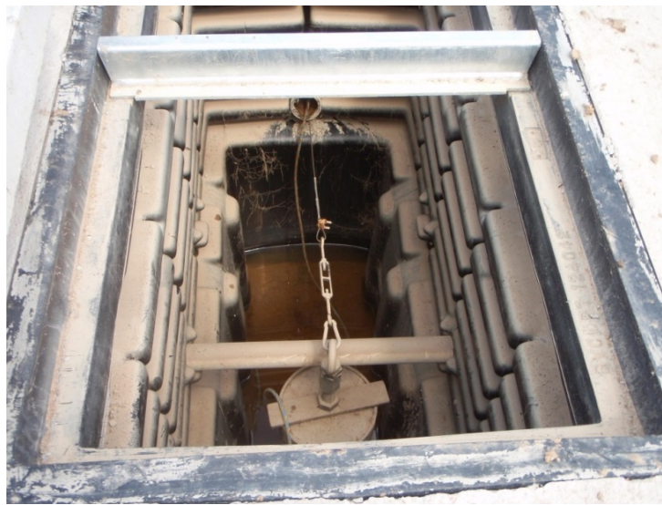
Figure 78 – Water at bottom of pit in WE2 anchor
