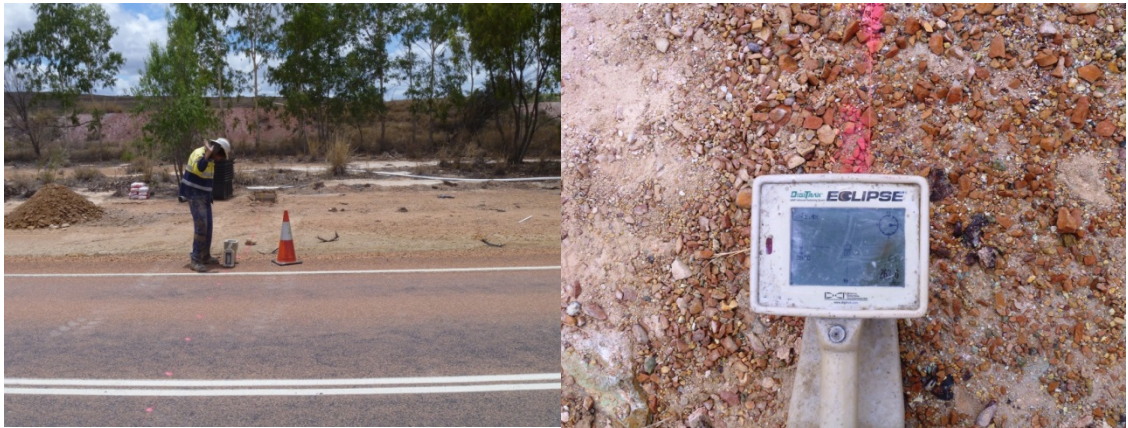
Figure 49 – Controlling drill position with location device
