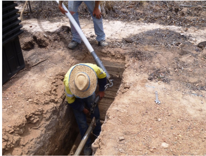
Figure 50 – Attaching conduit to drill for pulling through borehole
