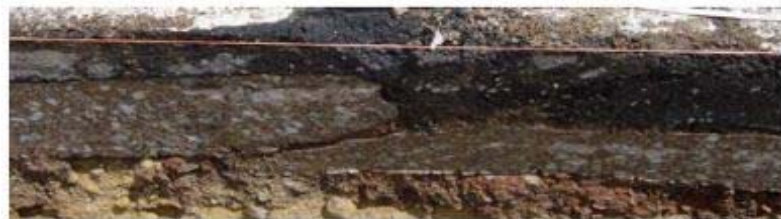
Figure 24 – Stepping in pavement surface caused by compressive strains (Nosenzo et al. 2013)
