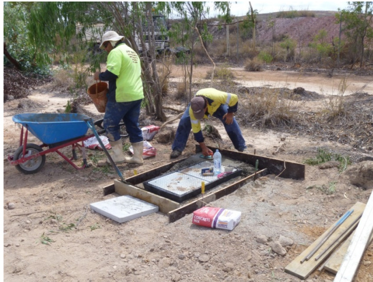
Figure 53 – Concreting pit surrounds
