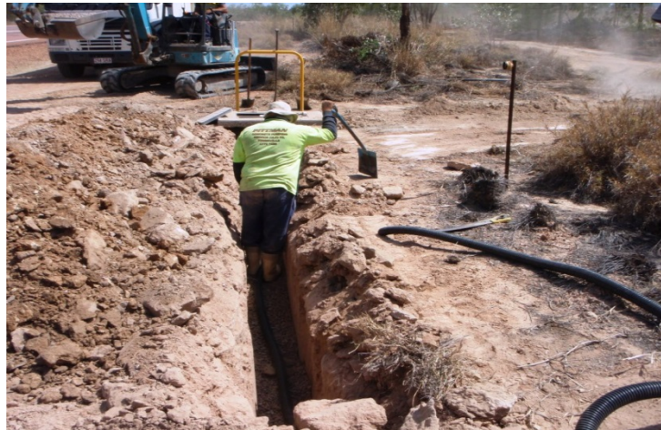
Figure 56 – Drainage trench for live end of pit
