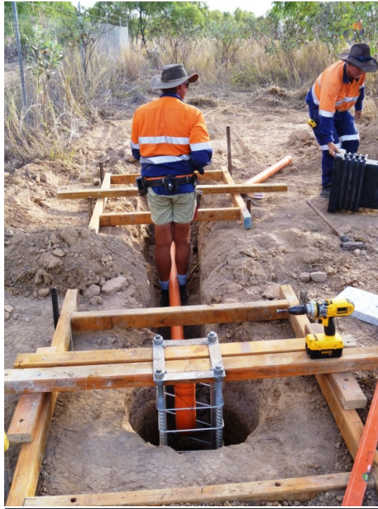
Figure 57 – Foundation formwork and reinforcement cage for communications pole
