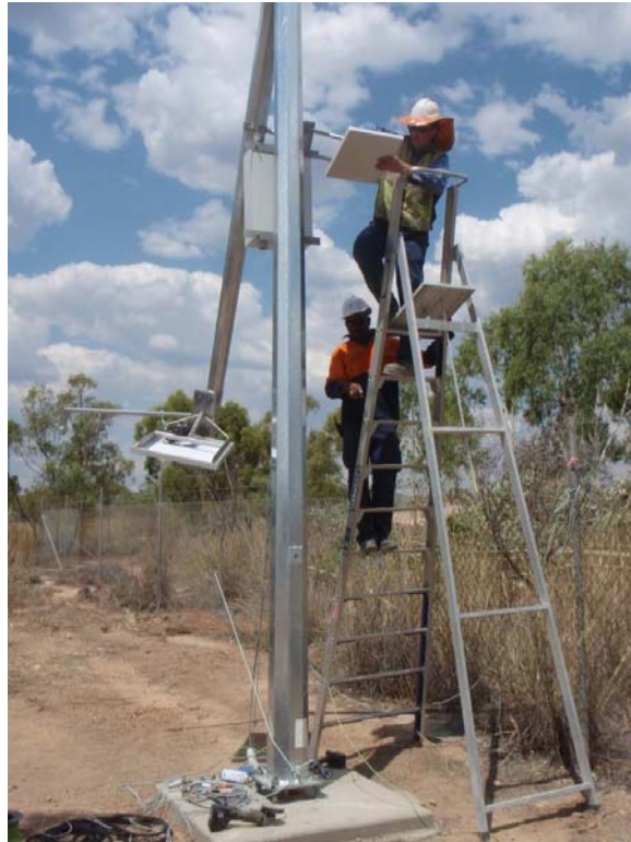
Figure 63 – Connection of satellite antenna to bracket
