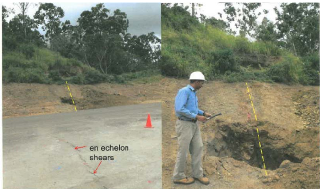
Figure 8 – Shear cracking in pavement and batter at Cut 3 after heavy rainfall (Starr et al. 2010)
