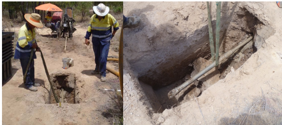
Figure 48 – Centralising drill through pit
