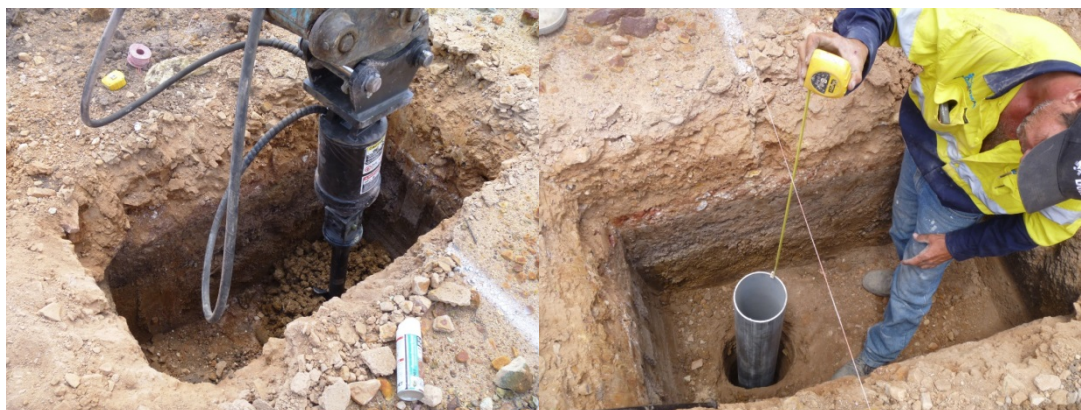
Figure 52 – Augering and installation of bollard
