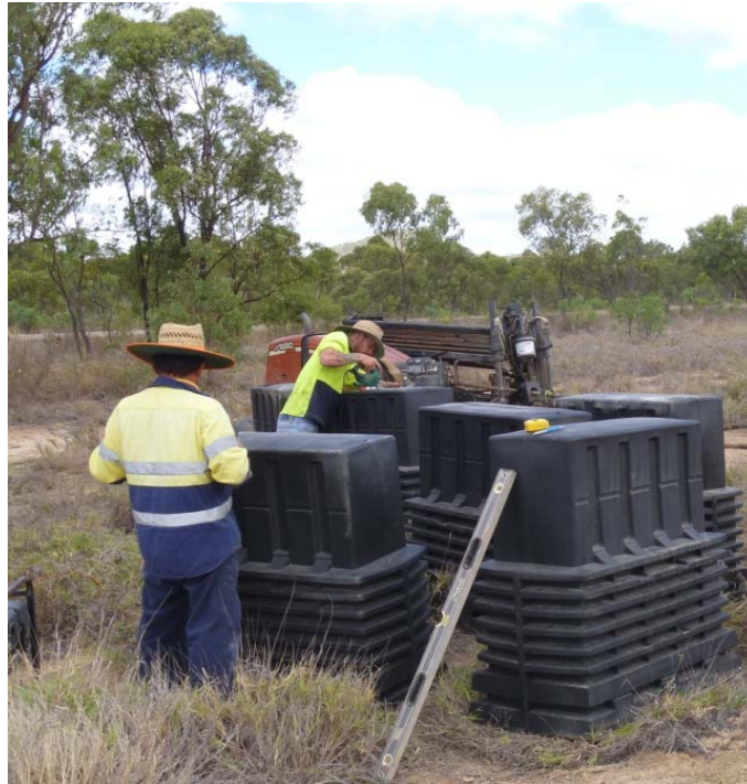
Figure 51 – Cutting base from bottom of pits
