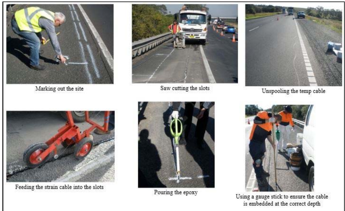
Figure 26 – Installation steps (Nosenzo et al. 2013)
