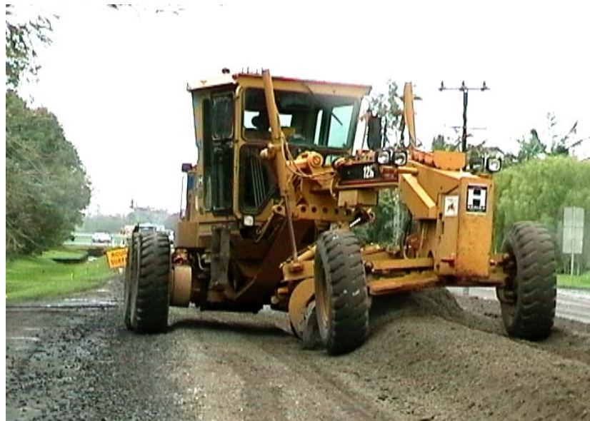
Figure 3.0 Grader trimming stabilised material
