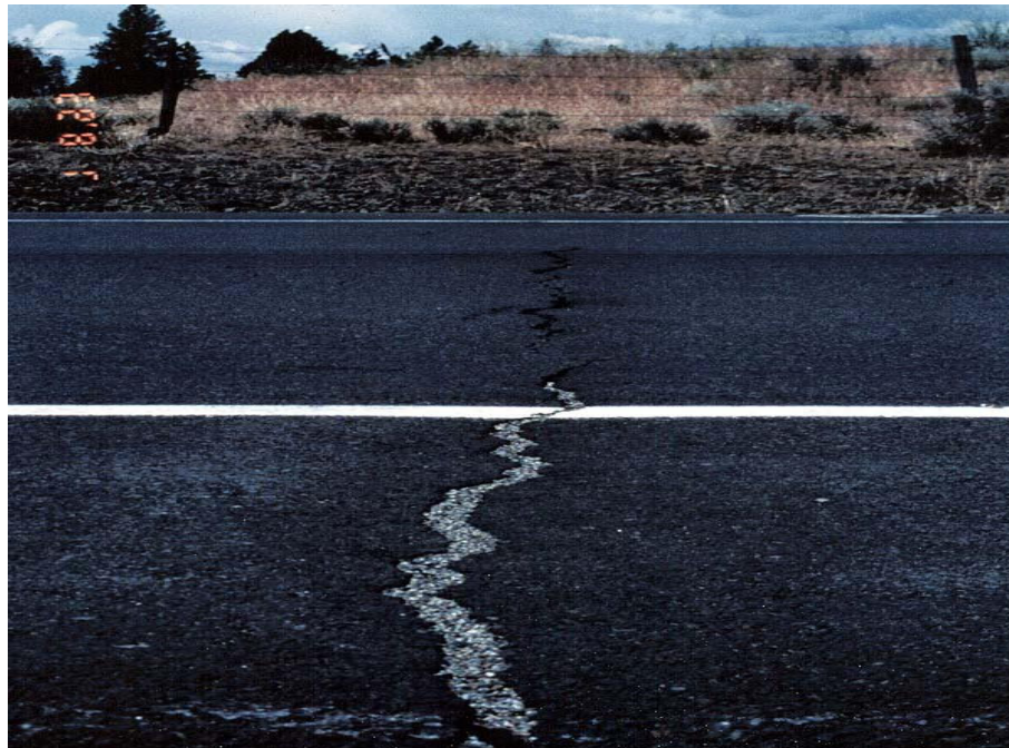
4.2.8 Transverse Cracking.
