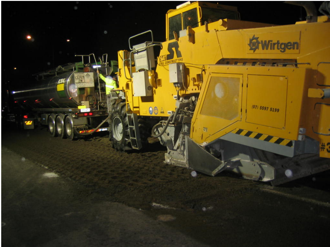
Figure 3.2 Foamed Bitumen Stabilisation
