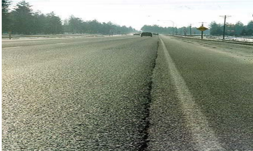
Figure 4.2.7. Longitudinal Cracking
