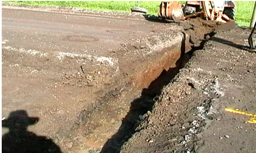
Figure 5.3 Pot Holing for soil sampling
