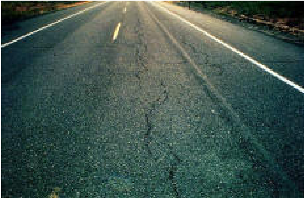
4.2.9 Meandering Cracks.
