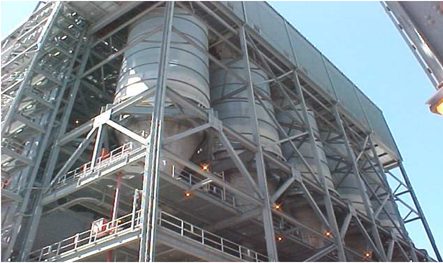
Figure 2-2: Coal Bunkers
