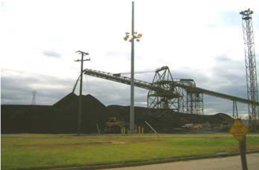
Figure 2-3 Coal transfer unit
