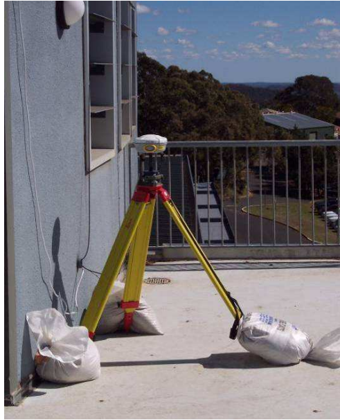
Figure 3.2.4 Receiver established next to wall on level 5 of Z-block.
