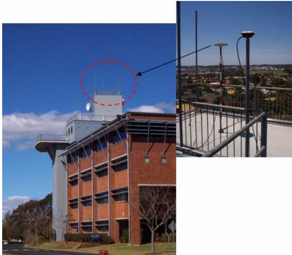
Figure 3.2.1 Level 7 base station.
