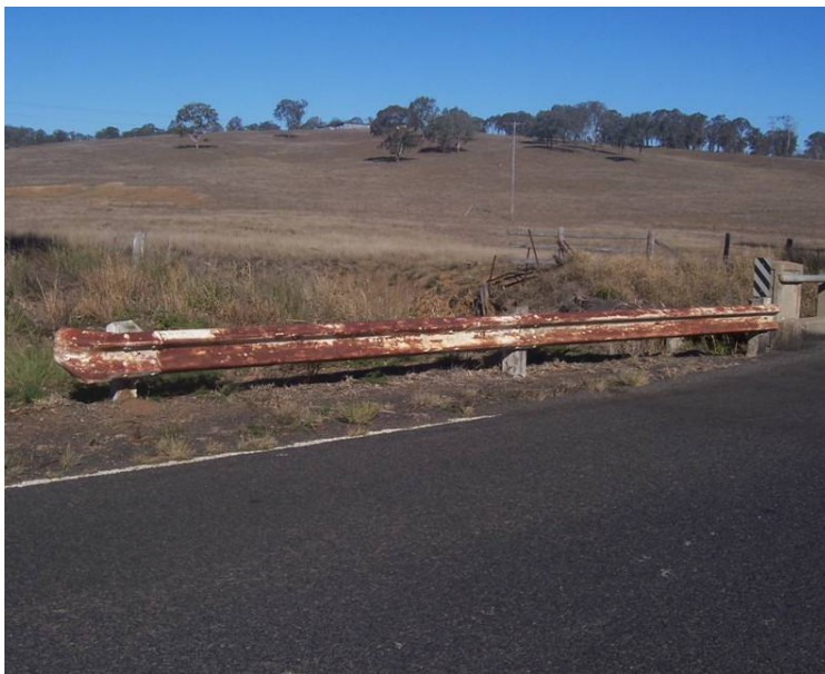
Figure 6-2 Photo of Murdering Hut Creek Guardrail
