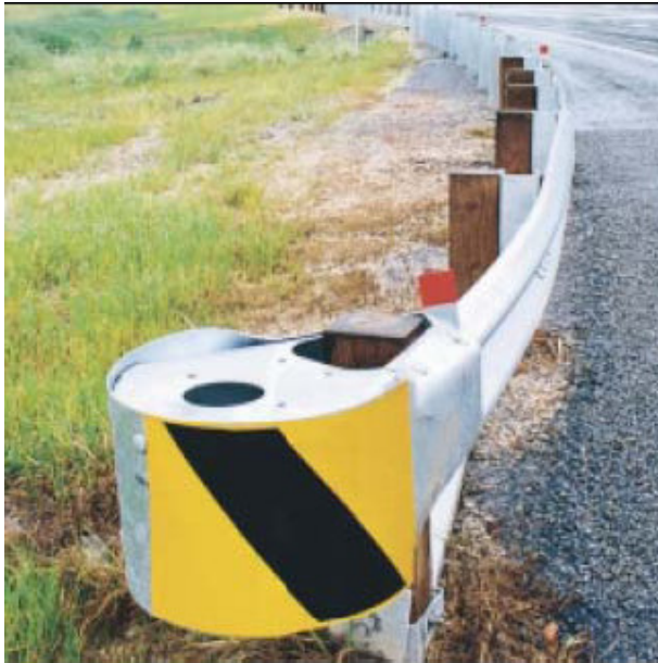
Figure 2-1 MELT (Modified Eccentric Loader Terminal) – Gating End Treatment Sourced (Vic roads 2005)
