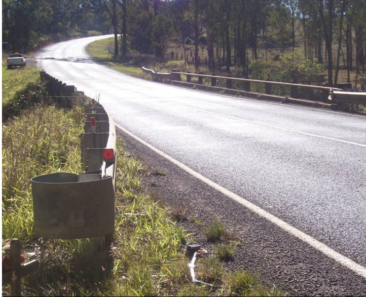
Figure 6-6 Photo of Rocky Creek Guardrail
