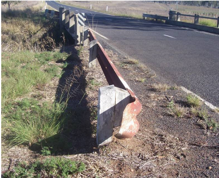
Figure 6-1 Photo of Murdering Hut Creek End Treatment
