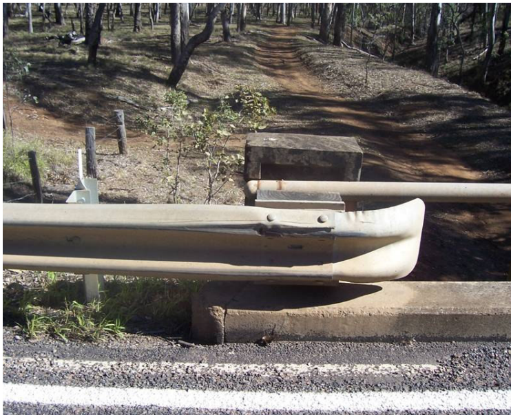
Figure 6-7 Photo of Rocky Creek Transition
