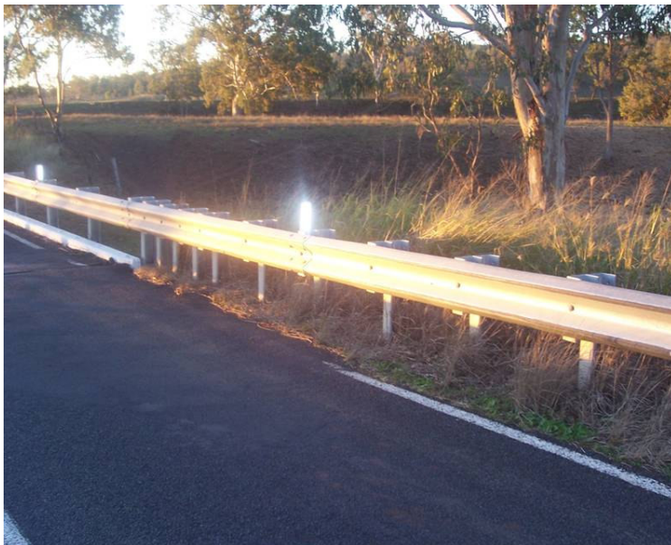
Figure 6-11 Photo of Kratzman's Gully Transition
