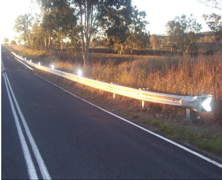
Figure 6-10 Photo of Kratzman's Gully Guardrail
