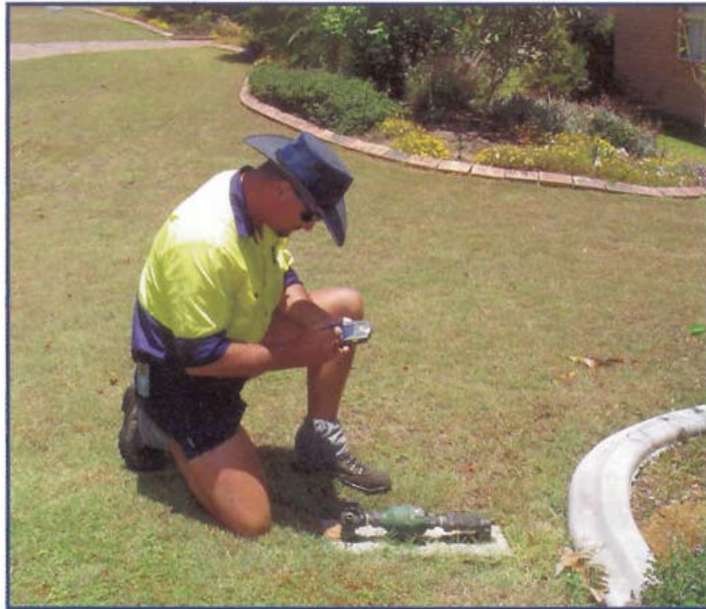
Figure 2.9 Meter reading with small handheld computers (Queensland Environmental Protection Agency and Wide Bay Water Corporation, 2005).
