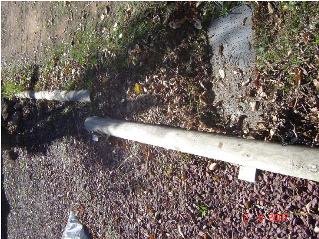
Figure C4 Property owners covering the water meter (copper logs for garden)
