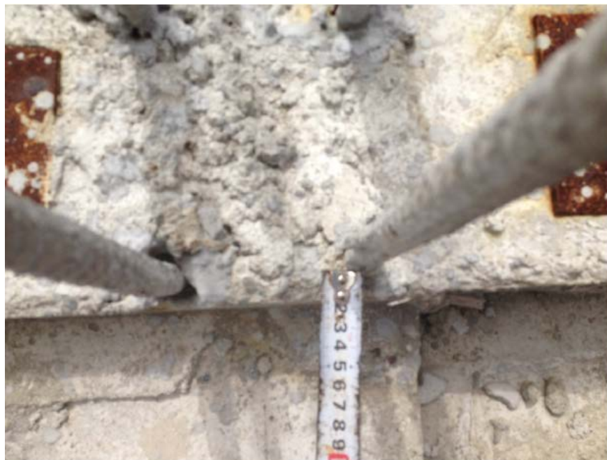
Figure 23: Shows 15mm Cover to Main Bar. Note the Bar Next to the One with the Tape Has Even Less Cover (NRW Macallan)
