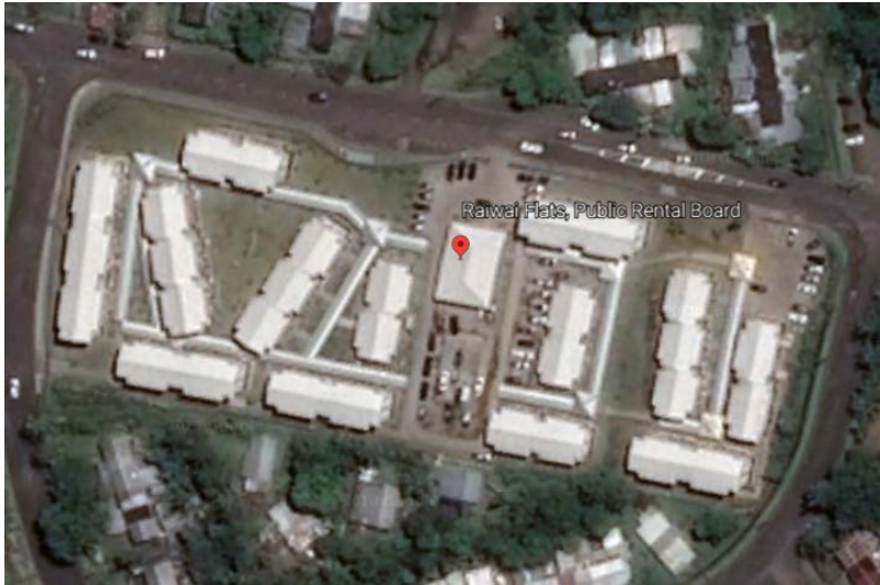
Figure 20: Shows an Aerial Photograph of the Site. (NRW Macallan)
