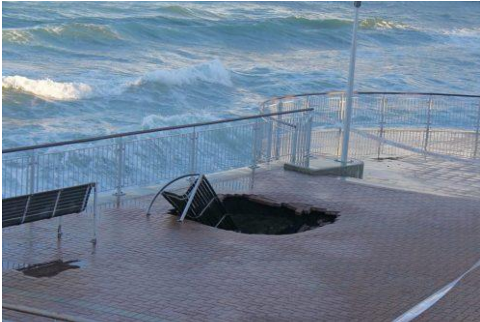
Figure 5, Sink Hole at St Clair Sea Wall
