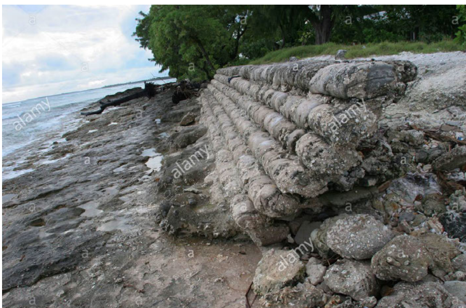
Figure 6, Broken and un-maintained sea-wall
