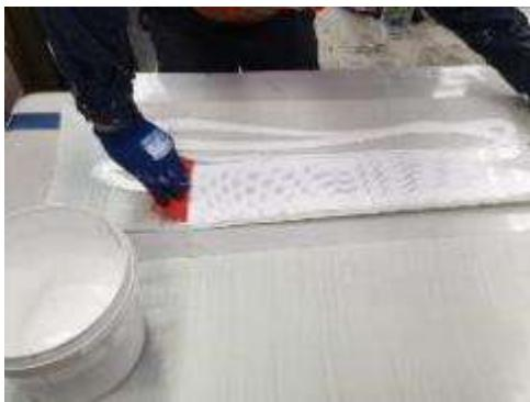
Figure 3-14 - Applying 220UR to FRP
