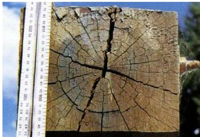
Figure 2-1 - Splitting due to thermal expansion (Bridge Inspection and Maintenance Manual 2001)
