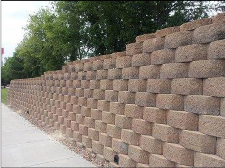
Figure 23: A typical segmented block wall (Dallas Fortworth Retaining Walls 2013)
