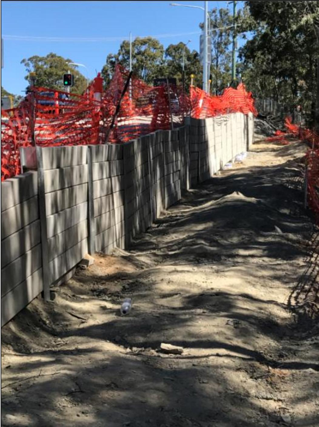
Figure 29: Gold Coast wall evidencing poor workmanship
