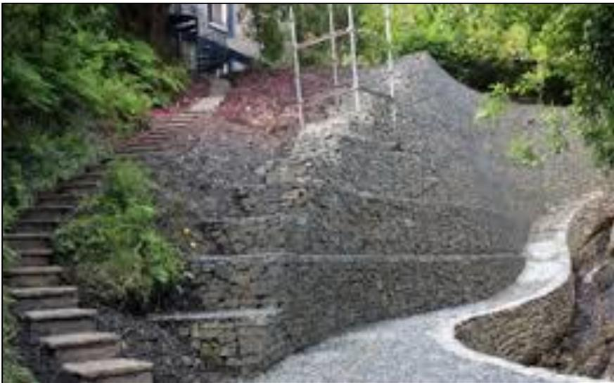
Figure 24: Large gabion wall in a residential setting (Fine Mesh Metals 2002)
