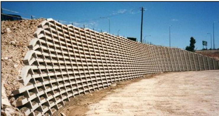
Figure 22: Crib wall at a height of approximately 4m high (Retaining Solutions 2017)
