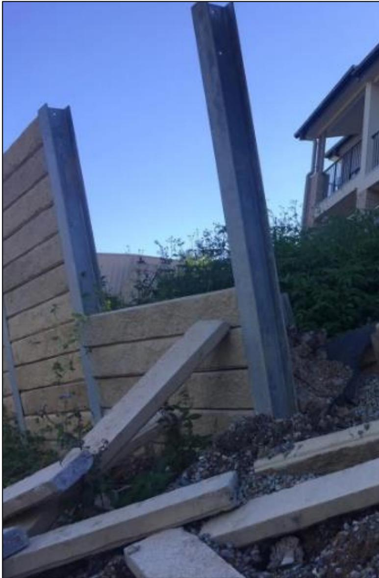
**Figure 27: Gold Coast wall failure (Brisbane Times 2017)**
