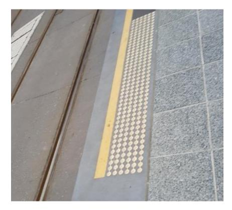
Figure C61. Yellow line tactile ground surface indicators.
