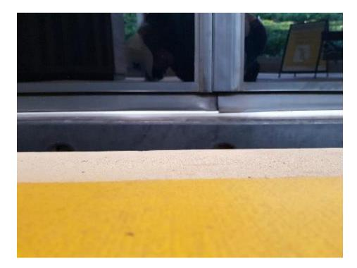
Figure 4.15. Height difference between the platform and light rail vehicle.
