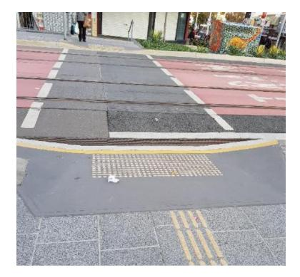
Figure C62. Tram track crossing with tactile surface indicators and yellow line.
