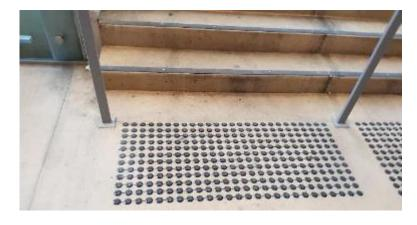
Figure C55. Tactile ground surface indicators at stairs.
