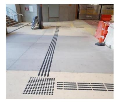
Figure 4.27. Tactile Surface Indicators.
