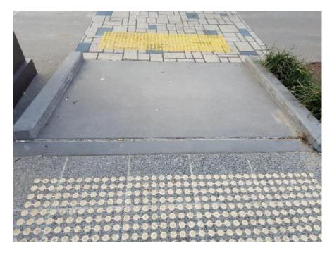
Figure C58. Tactile ground surface indicators at ramp.
