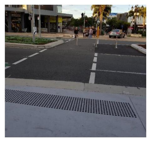
Figure C60. Signalised crossing and tractile ground surface indicators of kerb ramp.
