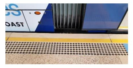
Figure C54. Yellow line tactile ground surface indicators.
