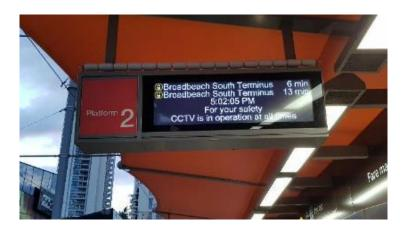
Figure C68. Overhead display of next two trams due on platform.
