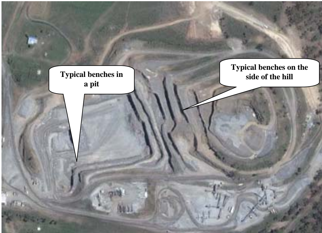
Figure 2.1 – Examples of Quarry Benches at Purga Quarry (Boral SEQ Quarries, 2006)
