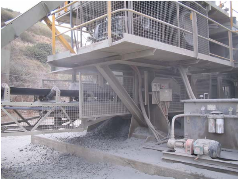
Figure 5.6: Platform that motor sits on at present
