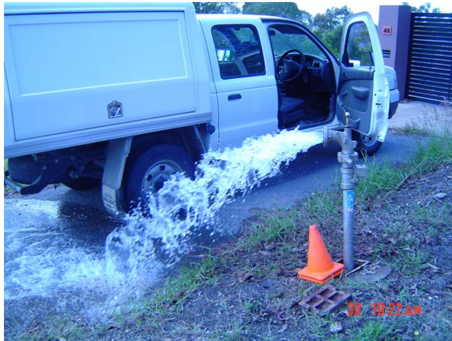
Figure 6.5: Hydrant being flushed downstream of Glenrowan Dr HLZ reservoir
