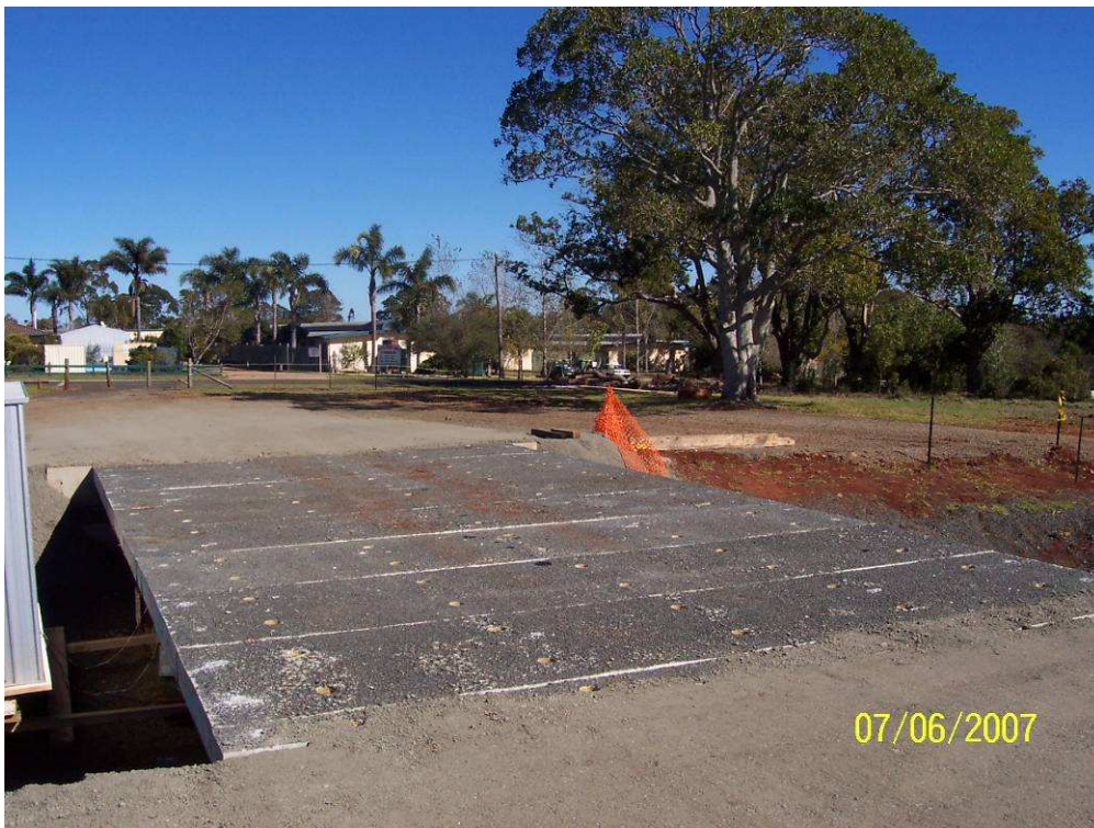
Figure B-3: Completed Bridge
