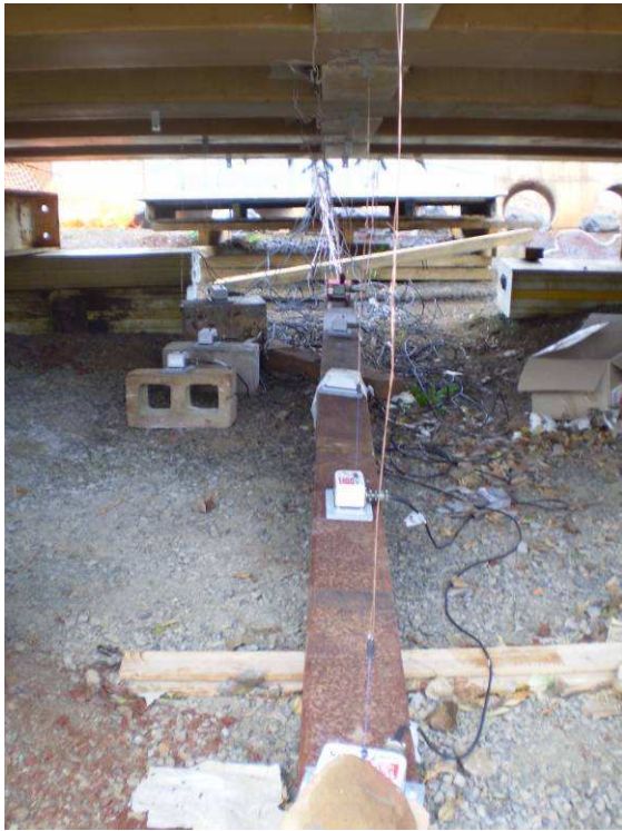
Figure 3-3: String pot positioning at girder mid-span
