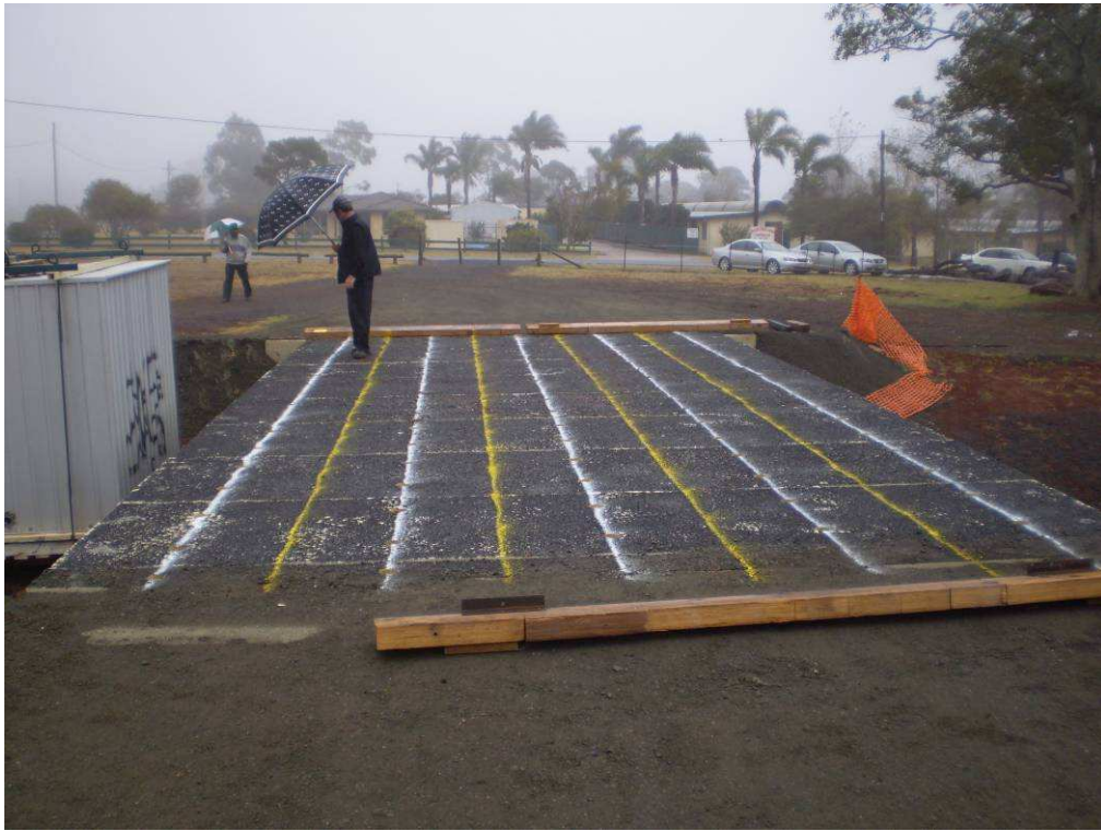
Figure B-4: Bridge marked for Testing Runs
