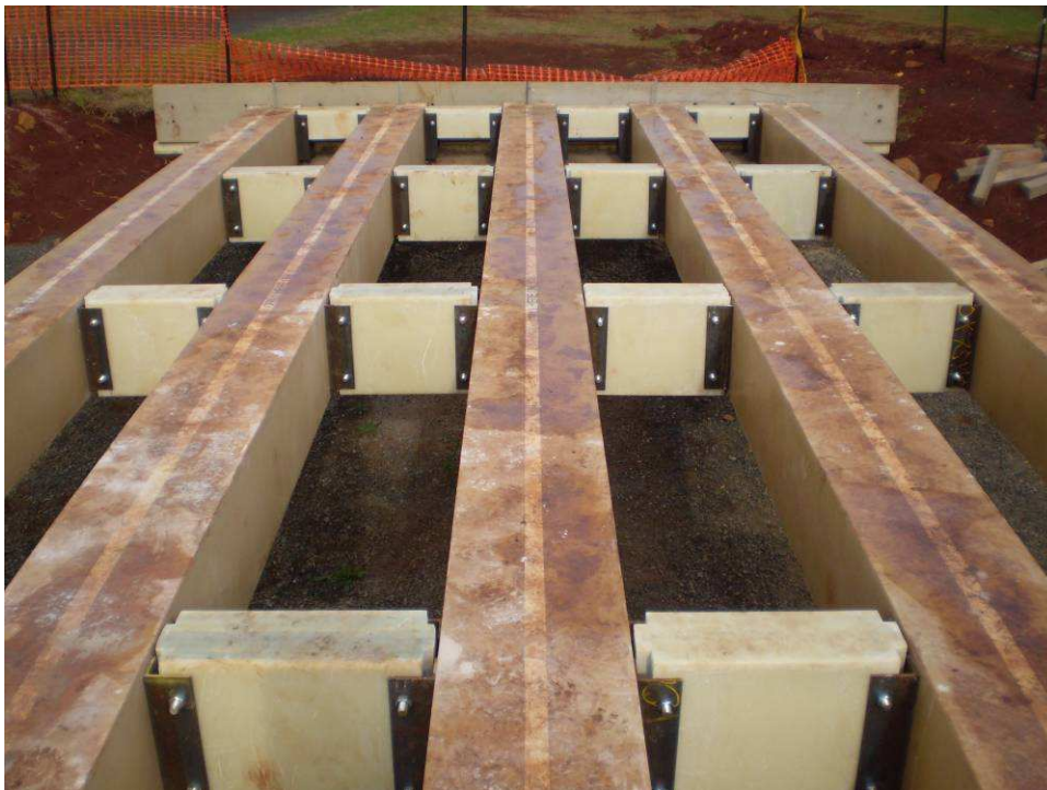
Figure B-1: Girder and Diaphragm Layout
