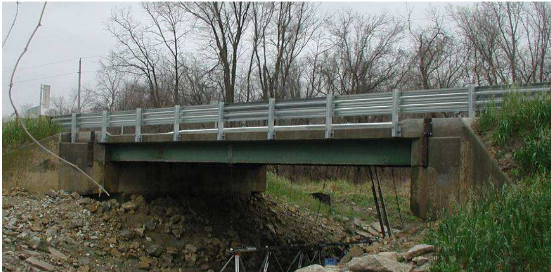
Figure 2-2: Elevation view of the Tama County Bridge (Dunn et al., 2005)
