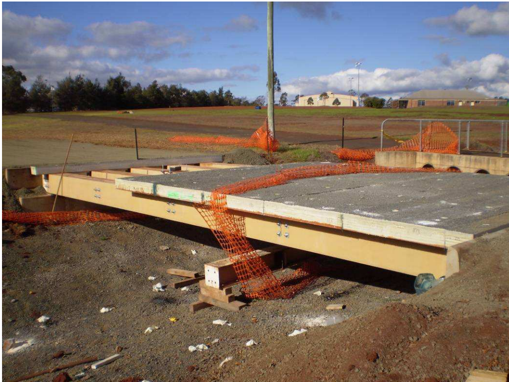
Figure B-2: Installation of Deck Panels
