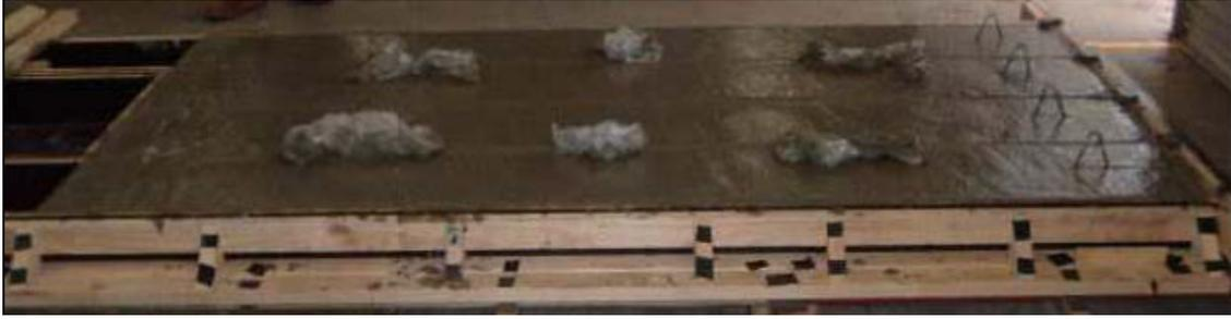
**Figure 4.1:** Beams after casting
