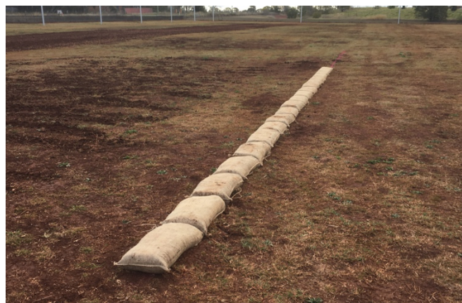
Figure 3.20: Sandbag berm
