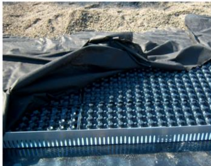
Figure 2.6 - Photo of Layers in a Green Roof System ( Magill, J., Midden, K., Groninger, J. and Therrell, M., 2011 )
