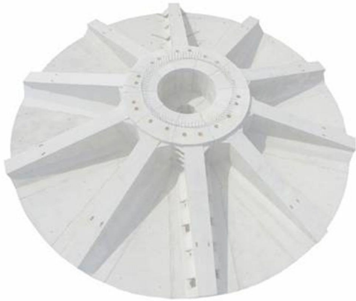
Figure 7. Precast wind turbine footing (Miceli, 2013)
