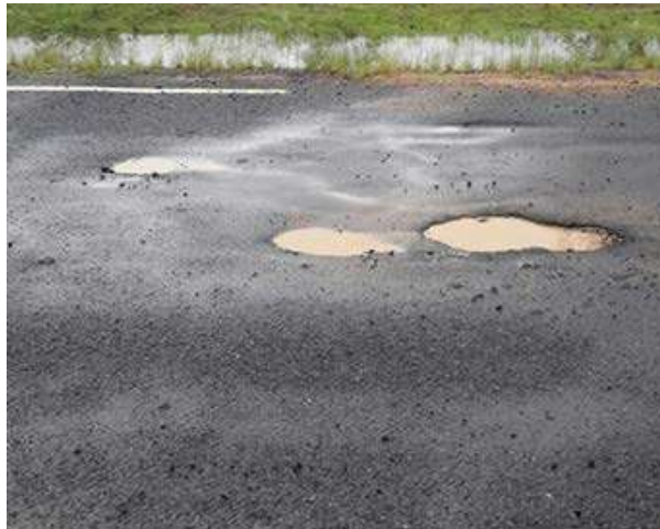
Figure 2.10: Potholes (TMR, 2017)
