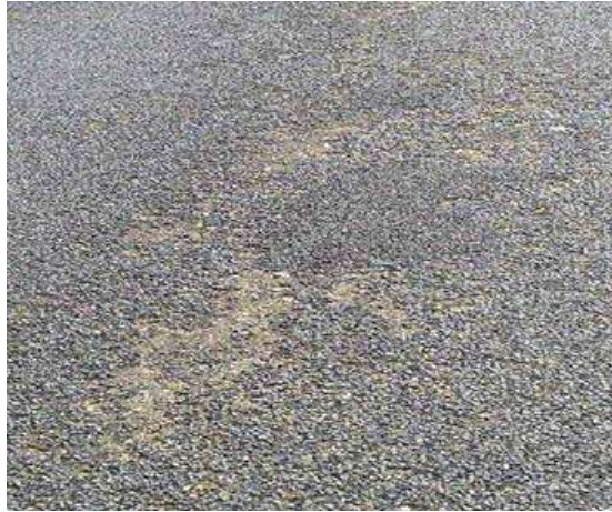
Figure 2.9: Stripping seal (TMR, 2017)
