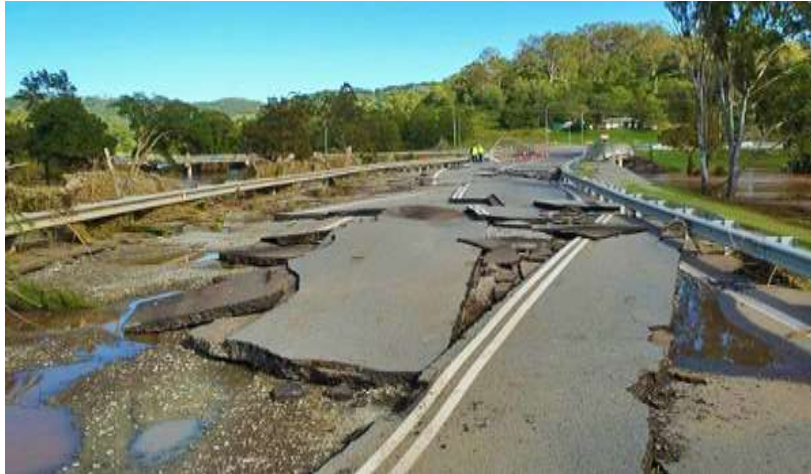
Figure 2.19: Alan Wilkie Bridge 2017 (CoGC, 2017)
