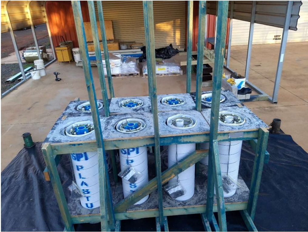
Figure 11: Specimens fixed vertically by the timber formwork prior to concrete placement
