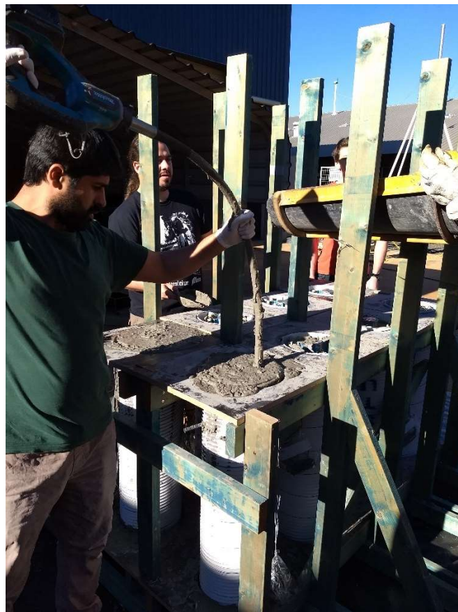
Figure 12: Electric vibrator used during concrete pour
