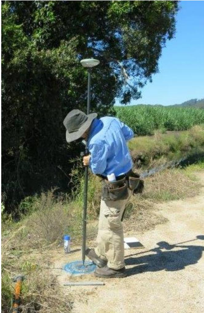
*Figure 19: Placement and GNSS observation of control points*
