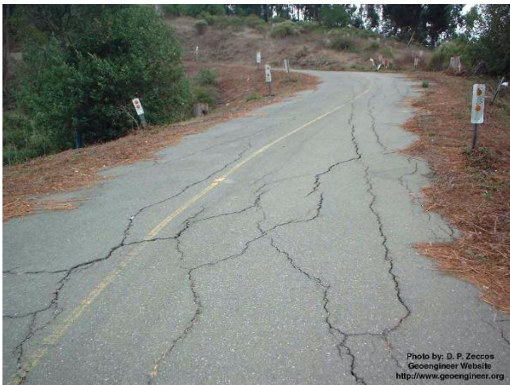
Figure 2-Cracking in pavement from swelling clay (Geoengineer.org 2018)
