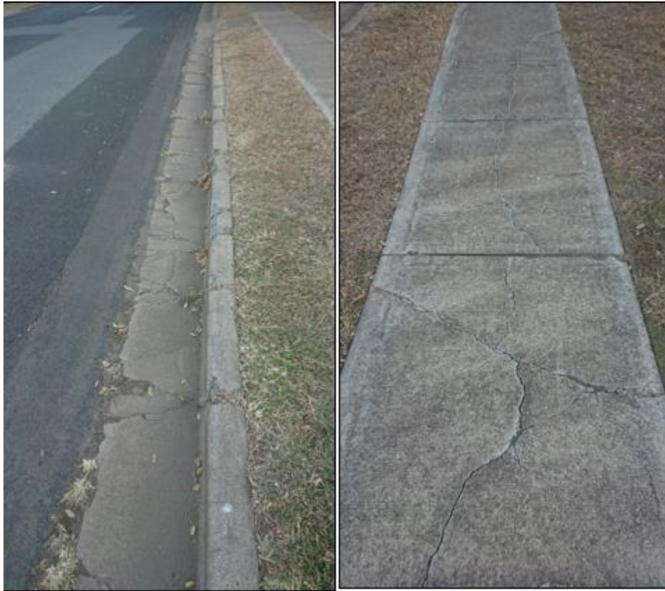
Figure 4-Cracking due to expansive soil Marburg QLD, (Author 2019)
