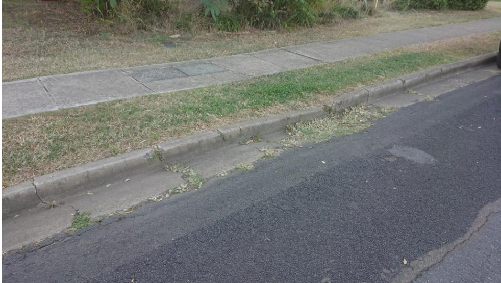
Figure 3- Pavement cracking due to expansive soil (Author 2019)
