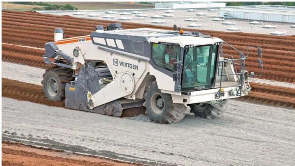
Figure 11- A soil stabiliser applying lime (Wirtgen 2019)
