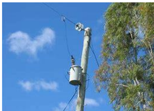
Figure 5.14 Single Wire Earth Return – SWER example (Source Ergon)
