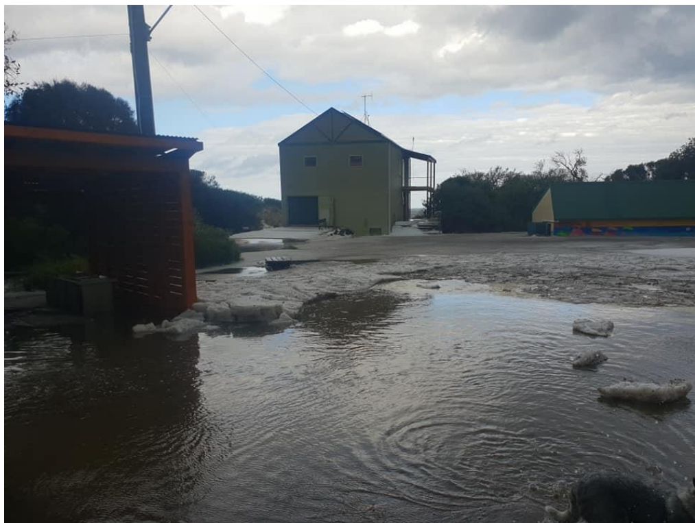
Figure 1.2: Flooding at Wonthaggi Surf Life Saving Club (Paterson 2019a)
