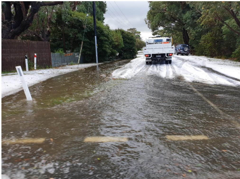
Figure 1.3: Localised flooding at Cape Paterson (Paterson 2019b)
