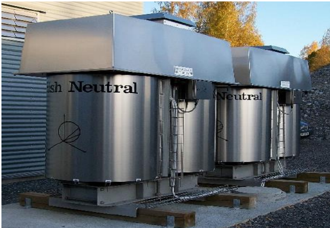
Figure 11: Arc Suppression Coils
