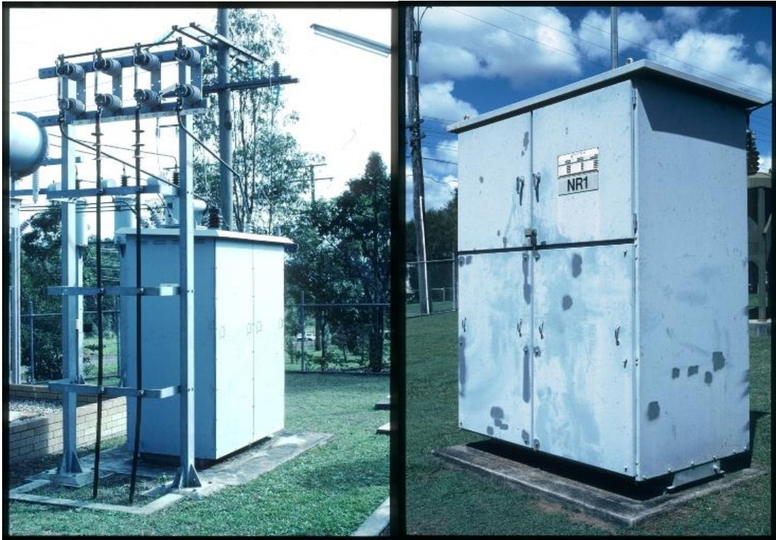
Figure 4: Neutral earthing resistor in field
