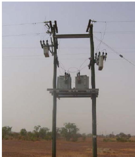
Figure 27: Duplex SWER System Configuration in Central Queensland
