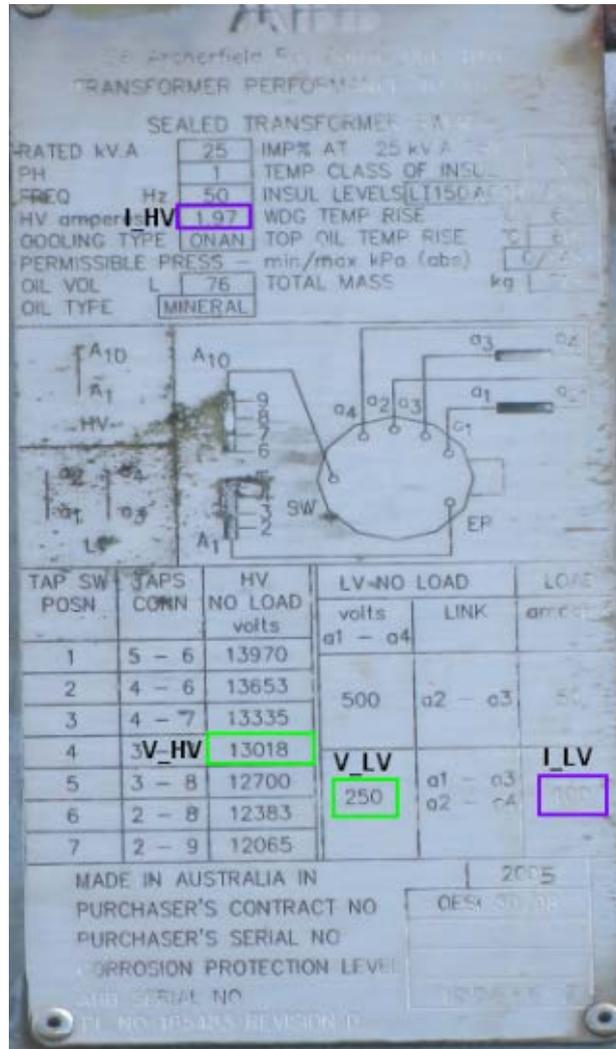
Figure 82: SS4631 Nameplate Ratings with HV and LV Values Highlighted
