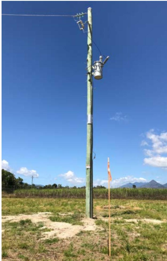
**Figure 120: Swallow Road Trial Site SWER Distribution Transformer SP806022**
