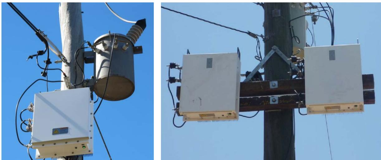
**Figure 29: LVR Units Fitted to SWER Distribution Transformers 240V and 480V Configuration**
