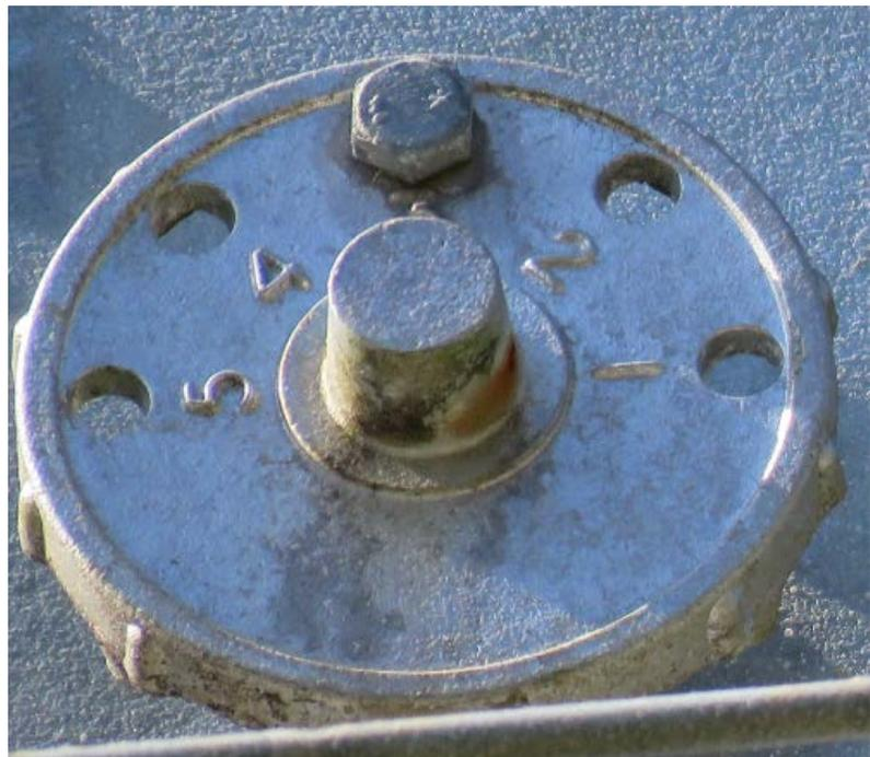
Figure 70: SS10620 SWER Isolating Transformer Nameplate and Tap Setting
