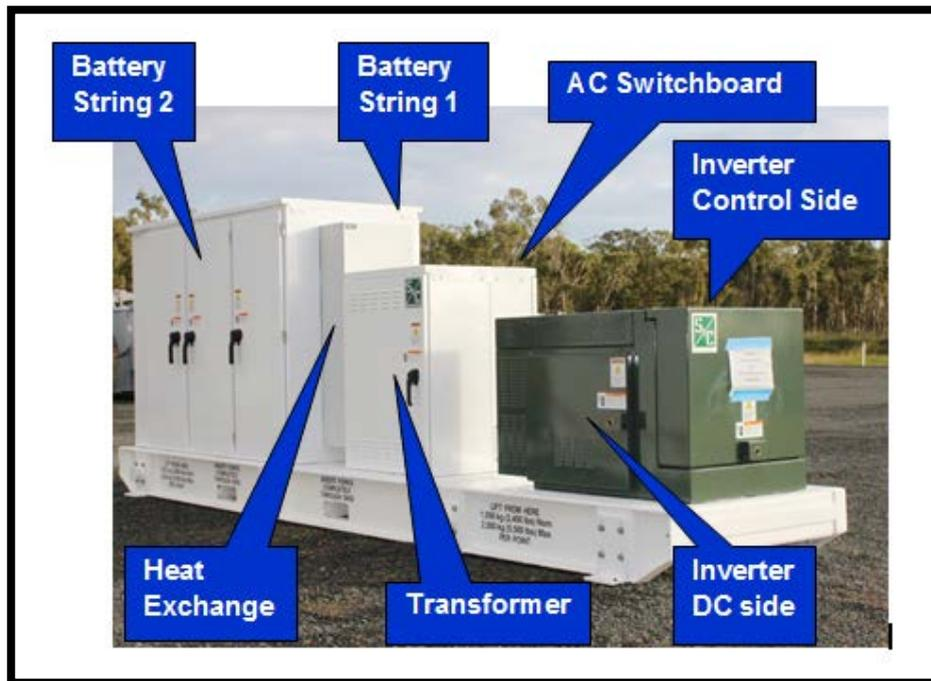
Figure 31: GUSS Unit Components (Ergon Energy 2019)
