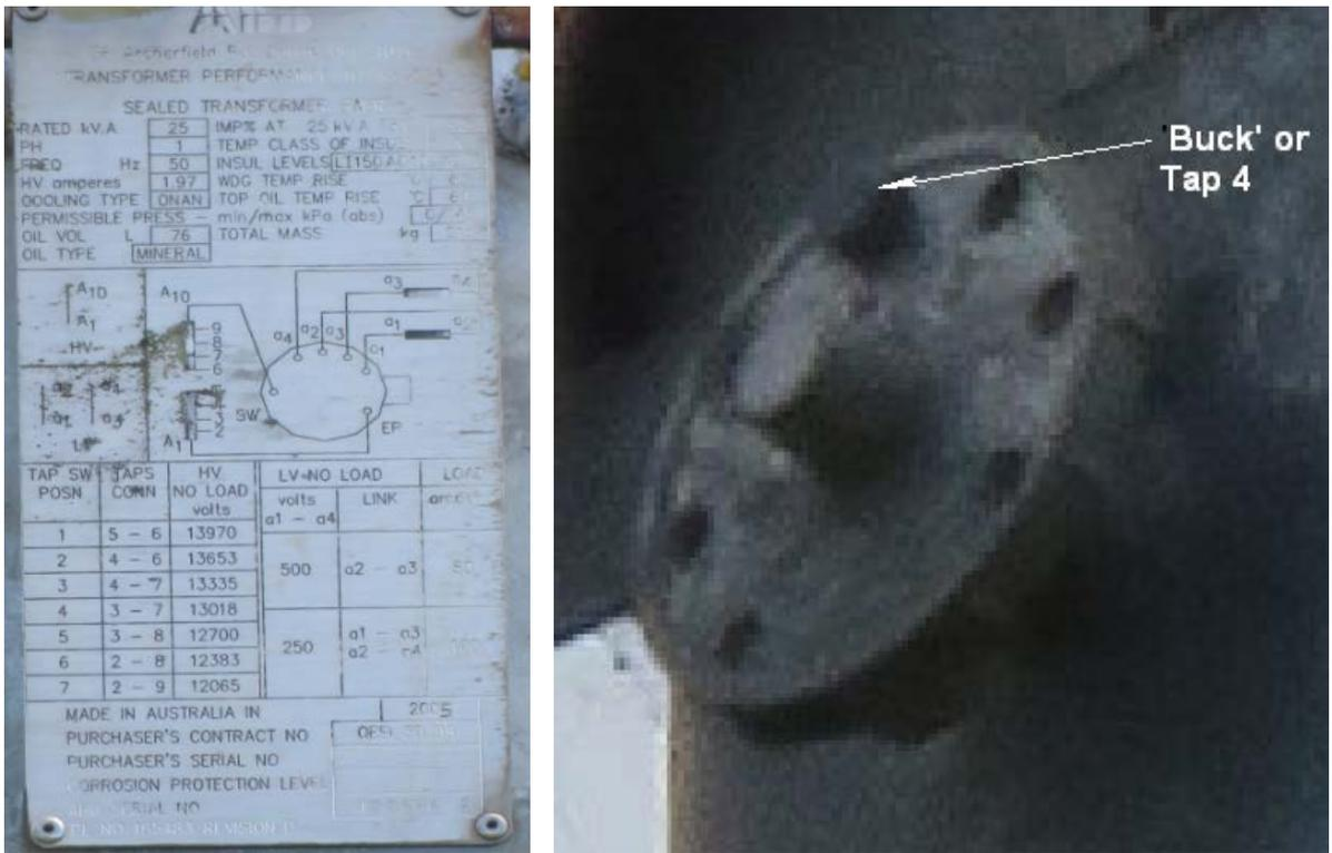
Figure 63: SS4631 Transformer Nameplate and Tap Setting
