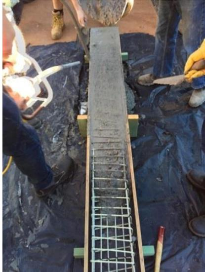
*Figure 4-6: Standard pouring methods were used to cast the sleepers*
