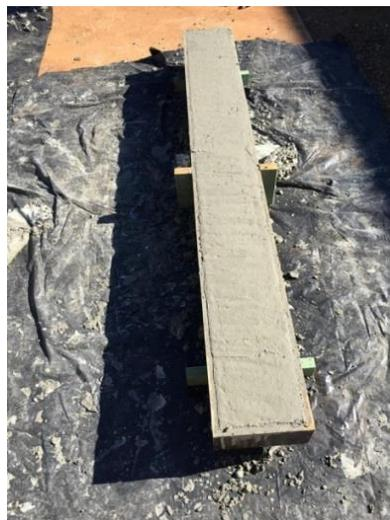
*Figure 4-7: Screeded sleeper in its precast mould*
