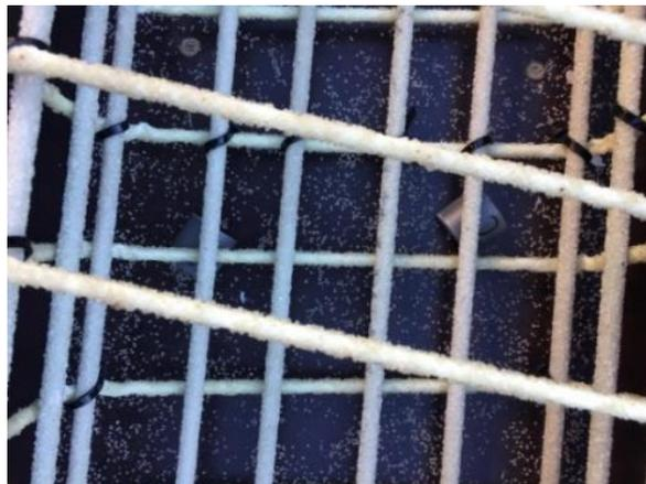
*Figure 4-2: Cable ties used to fix flexural and shear reinforcement together*
