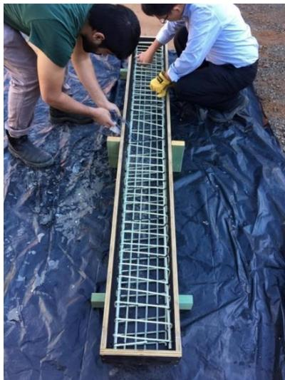
*Figure 4-4: The assembled reinforcement cage in the precast sleeper mould*
