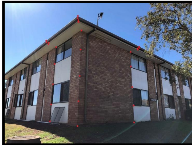
Figure 9 Points captured by the Total Station
