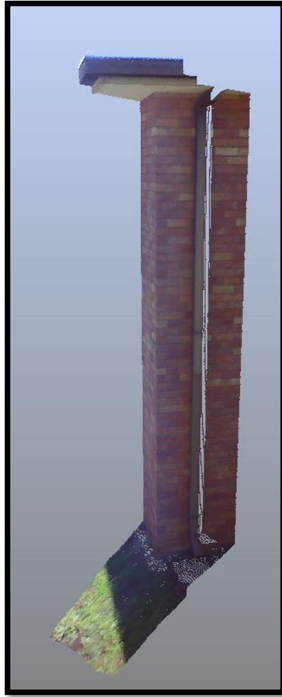
Figure 29 SW Building corner snippet from FARA Scene
