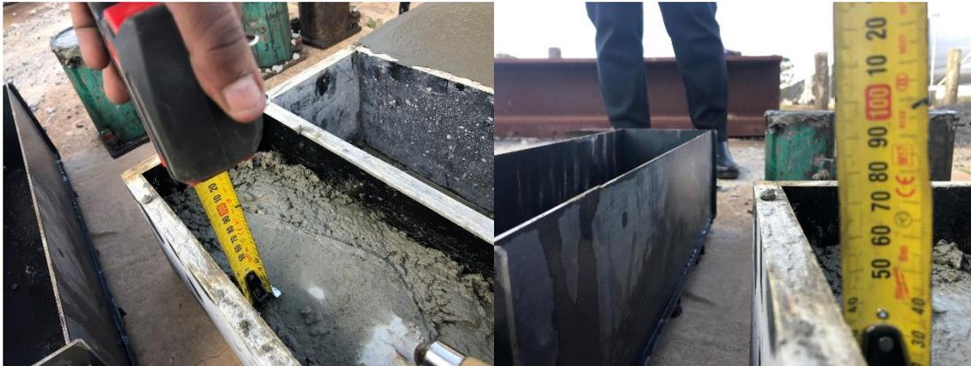
Figure 4.6: 40mm graphene/concrete moulding pictures
