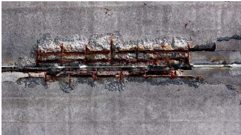
Figure 1: Reinforcement Corrosion in Concrete ( Markham, 2016 )
