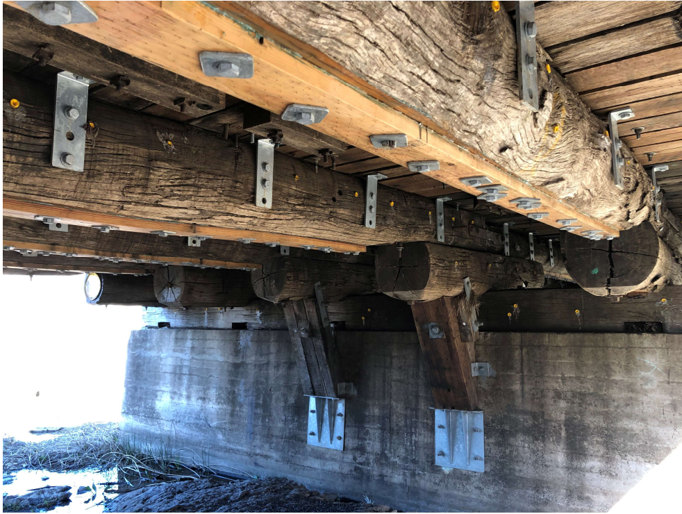
Figure 4: FRP Retrofit as Constructed
