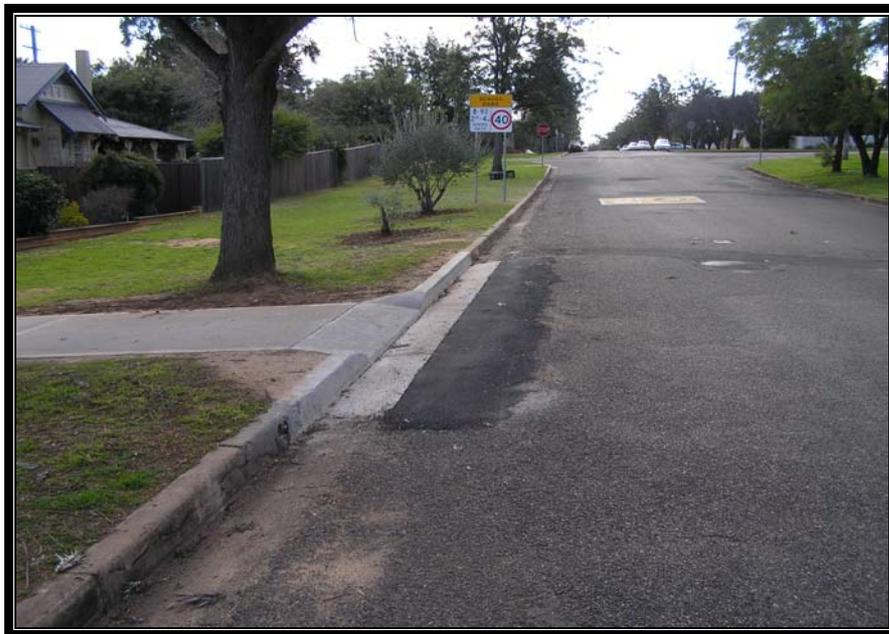
**Figure 7-2 – Realignment of existing kerb and gutter**
