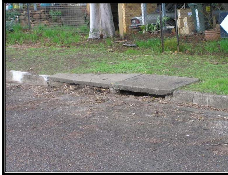
**Figure 5-4 – A typical inlet pit in East Tamworth**
