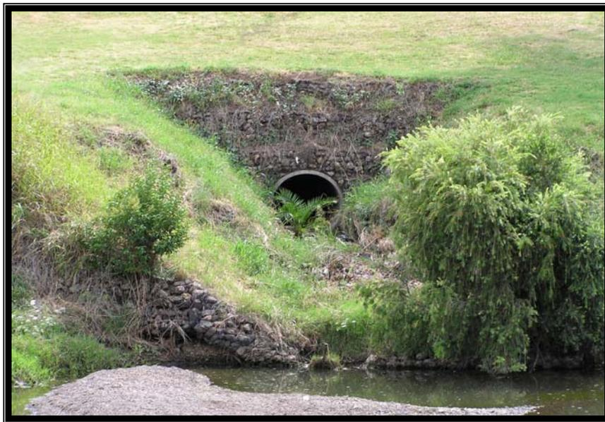
**Figure 3-3 – Pressure Drains Outlet Located at Fitzroy and the Peel River**
