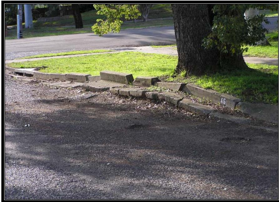
Figure 7-1 – Unaligned kerb and gutter in the East Tamworth area
