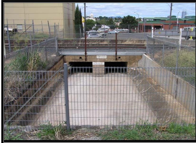
**Figure 3-2 – Pressure Drains Inlet Located at Fitzroy and Marius Street**
