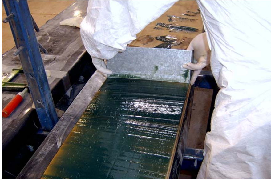
Figure 5.5 Glue being spread between LVL layers.
