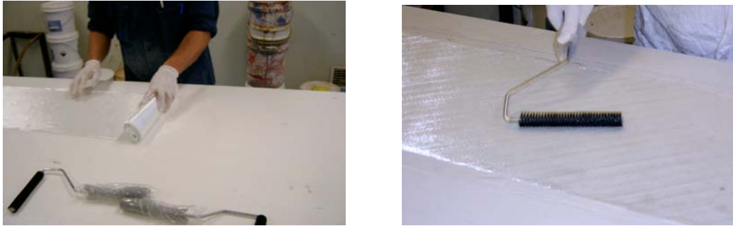
Figure 5.2 Resin coating of fabric in laminate panels.
