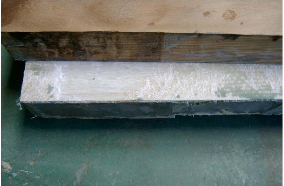
Figure 6.6 Failure of tension module.
