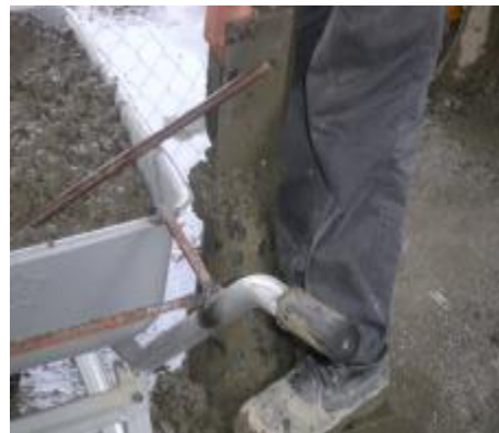
Figure 4.6: Fill in 3 layers and compact in standard manner.
