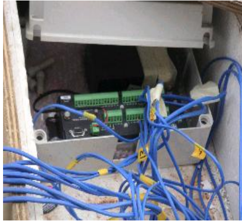
Figure 5.10: The thermocouple wires are numbered with yellow color tag.
