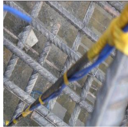
Figure 5.7: The additional steel bar was tied to the structure.
