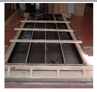
Figure 4.1: Formwork to Cast Beams
