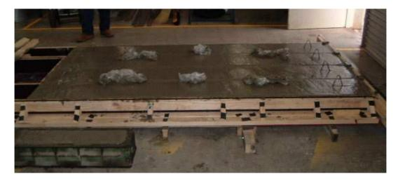
Figure 4.6: Freshly Cast Beams
