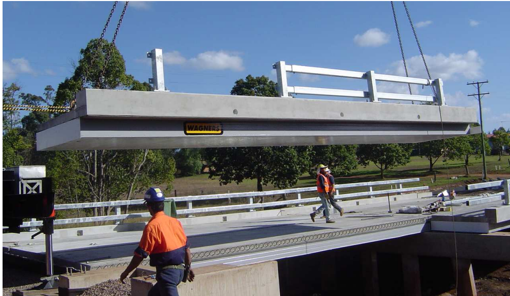
Figure 3.6: Picture of a Hybrid Concrete-FRP Bridge Deck Produced by WCFT
