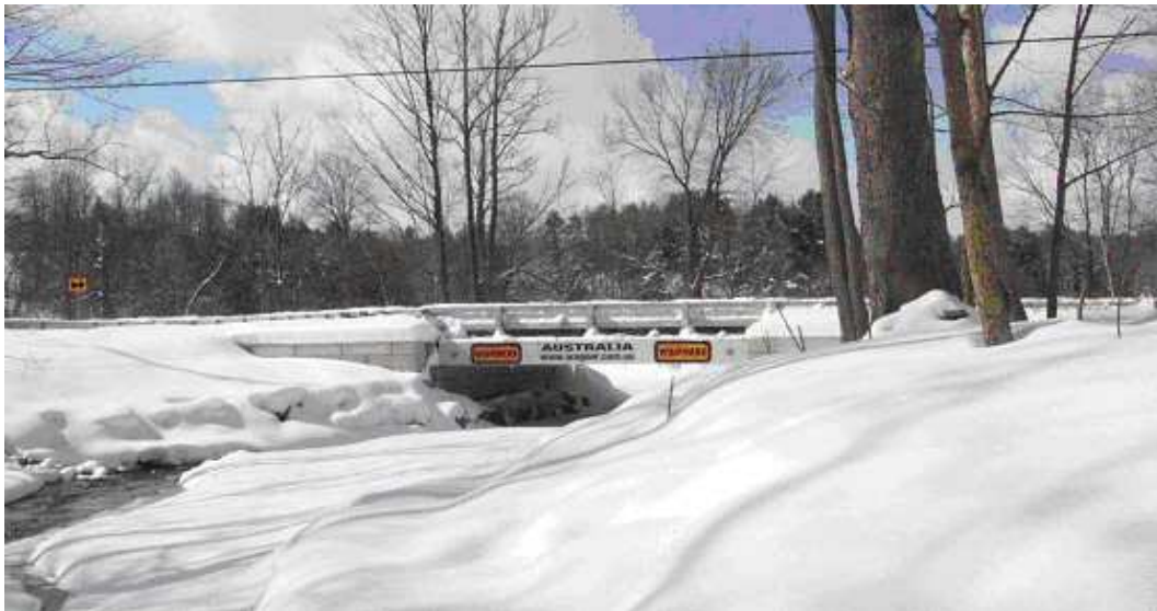
Figure 1.3: Wagner Composite Technologies Bridge Installed in Erie County, New York, United States of America (Source: [2])
