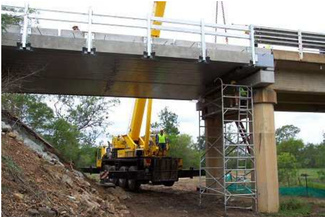
Figure 1.2: 1st FRP Bridge in the Australian Public Road Network (Source: [2])
