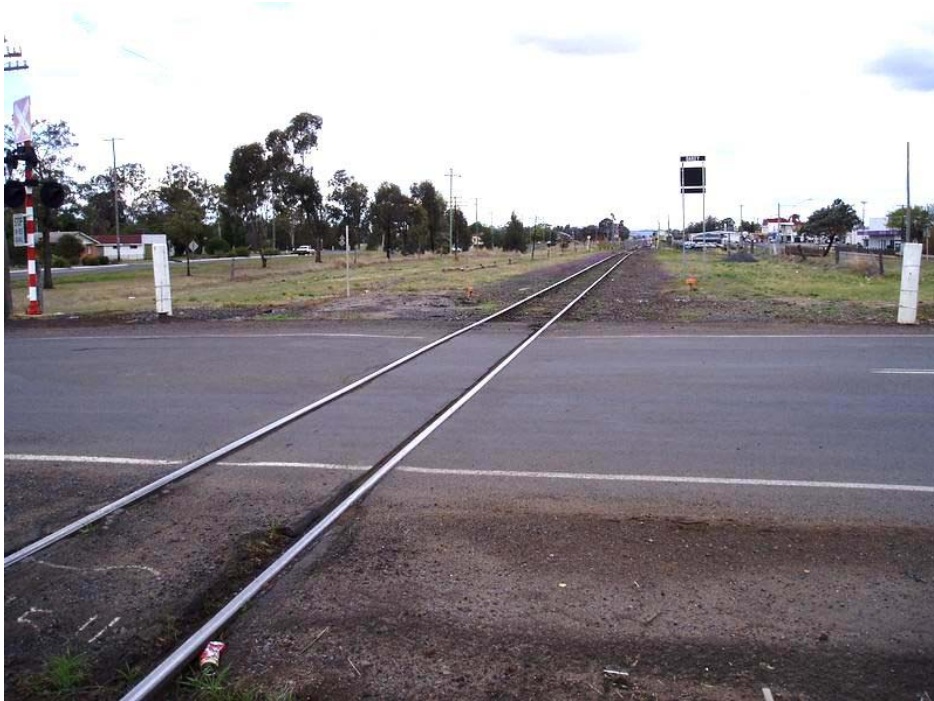
Figure 7.2b: Railway Crossing at the South End of 417
