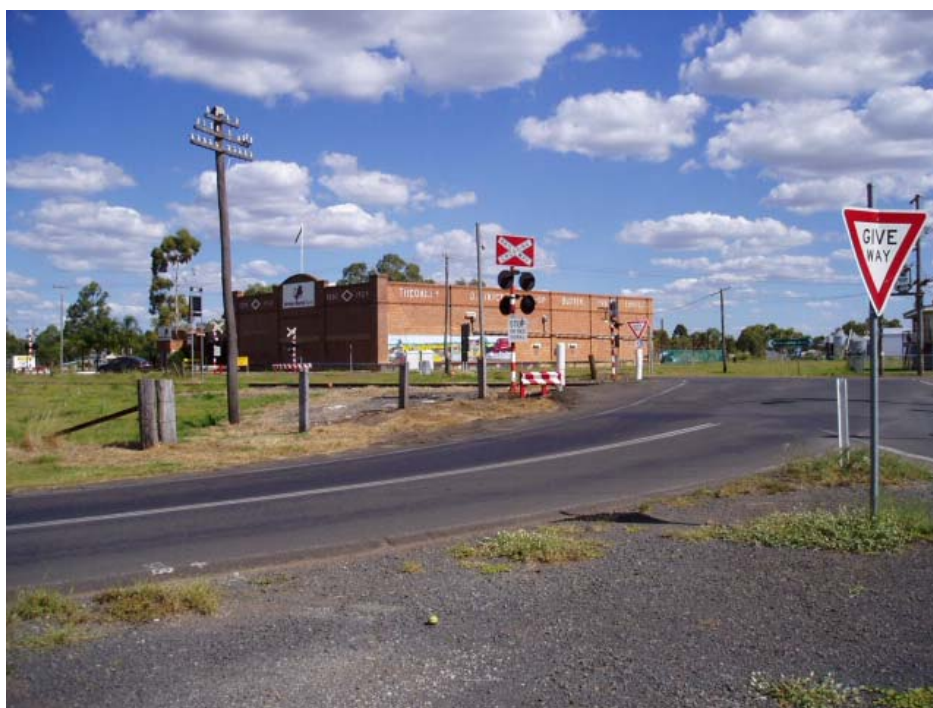
Figure 7.2a: Railway Signal at the South End of 417
