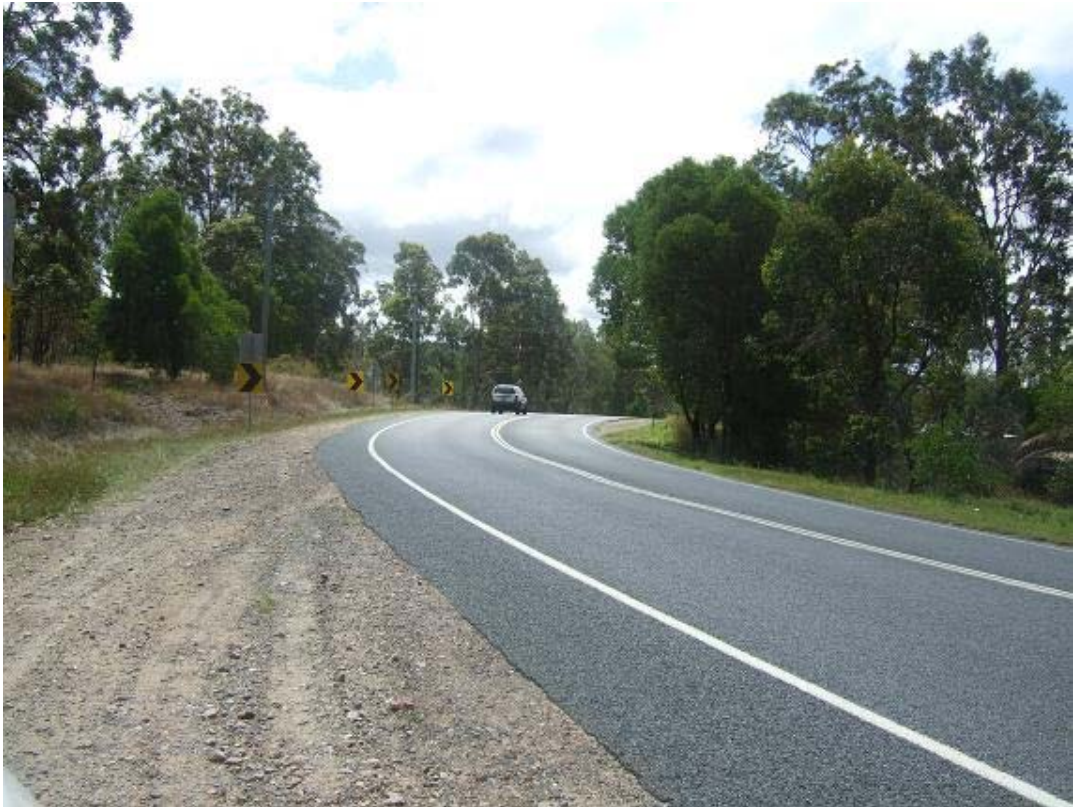
Figure 6.5 – Westbound Approach to Element 30
