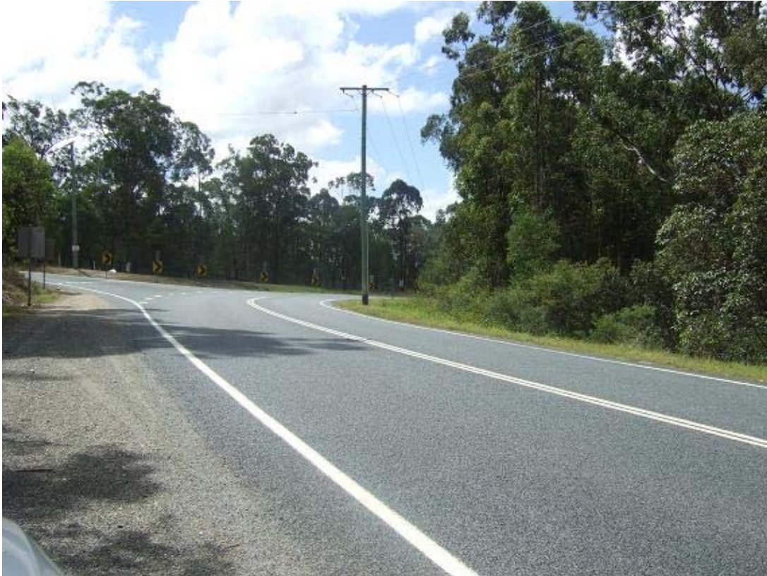
Figure 6.6 – Westbound Approach to Element 25
