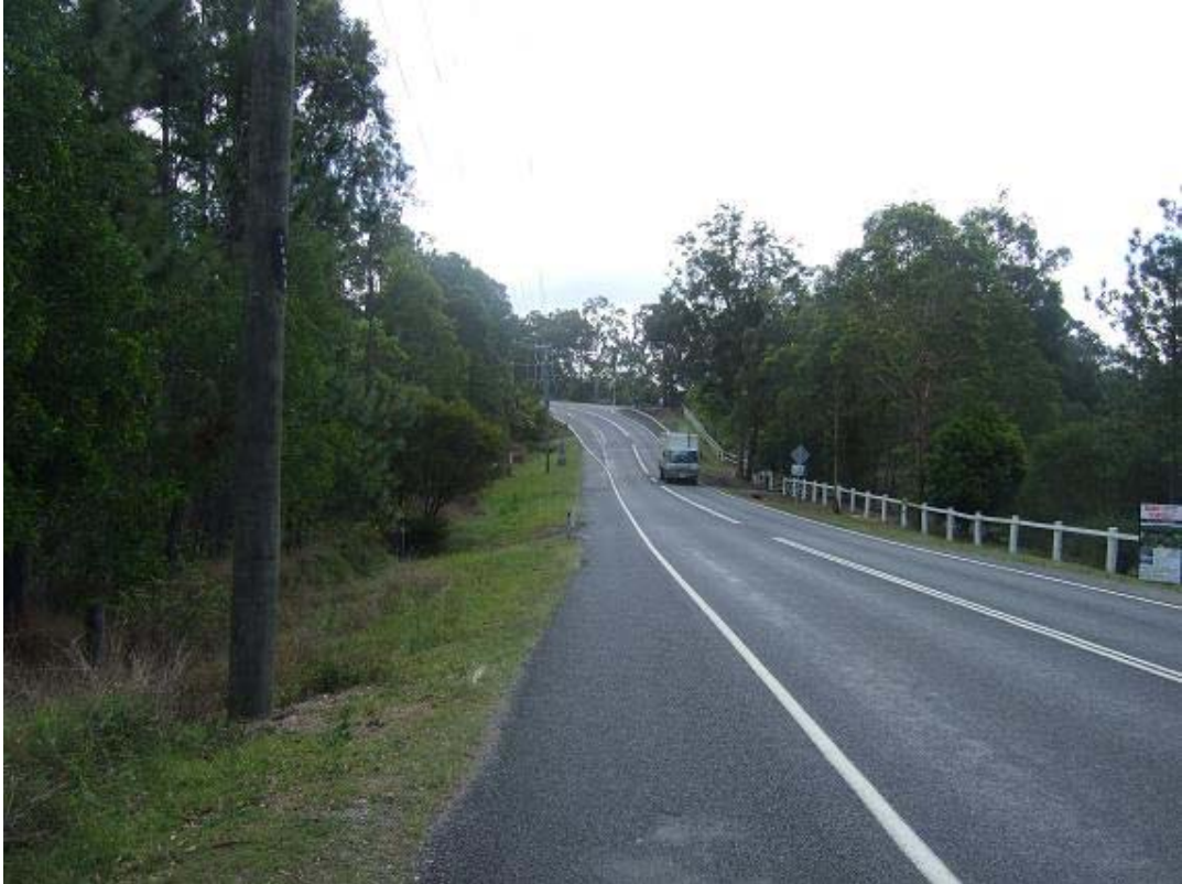
Figure 6.4 – Westbound Approach to Element 34
