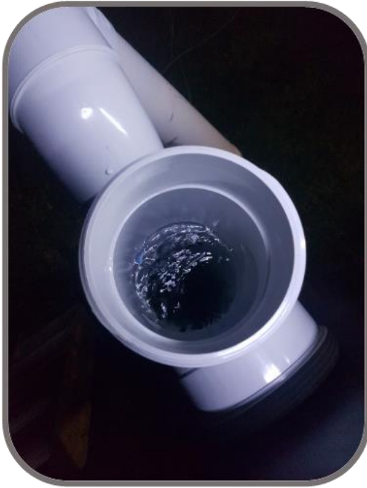
Figure 3.10: Inspection opening (A Brian 2021, personal photograph, 22 September)
