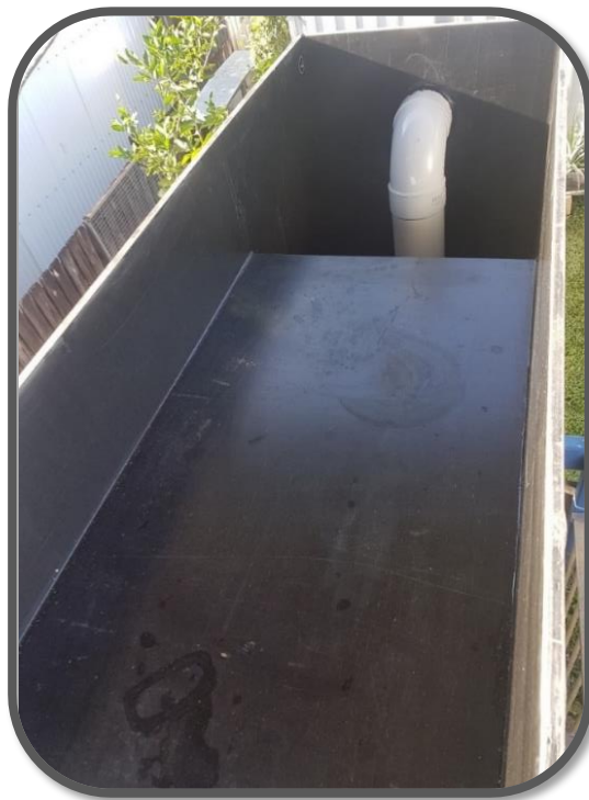
Figure 3.4: Containment area (A Brian 2021, personal photograph, 22 September)
