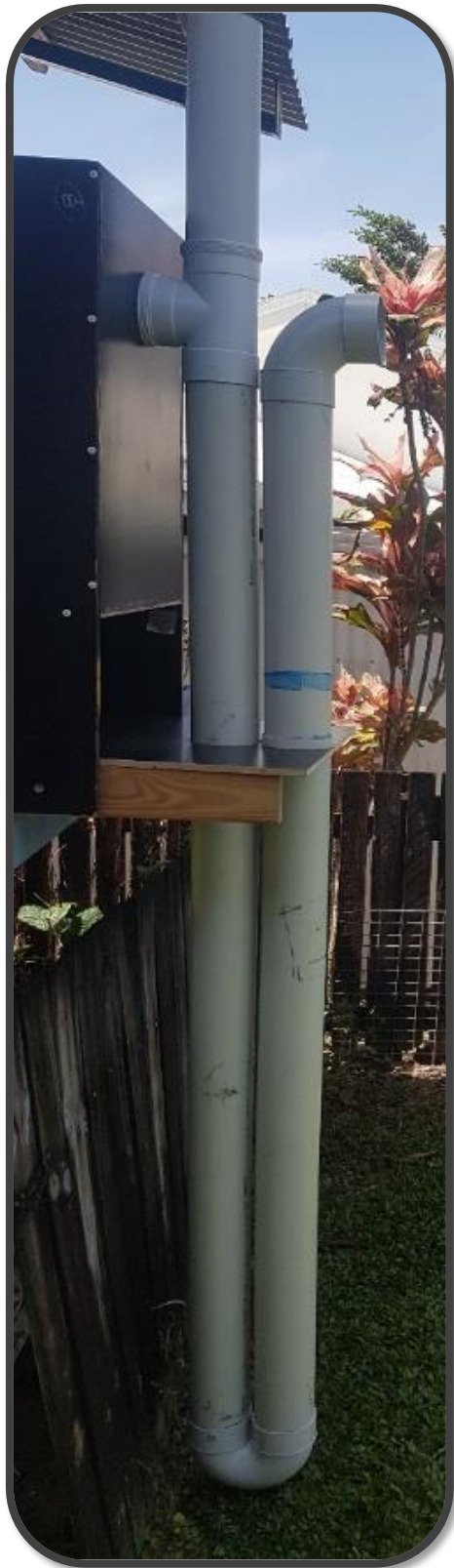
Figure 3.6: Constructed U-tube (A Brian 2021, personal photograph, 22 September)
