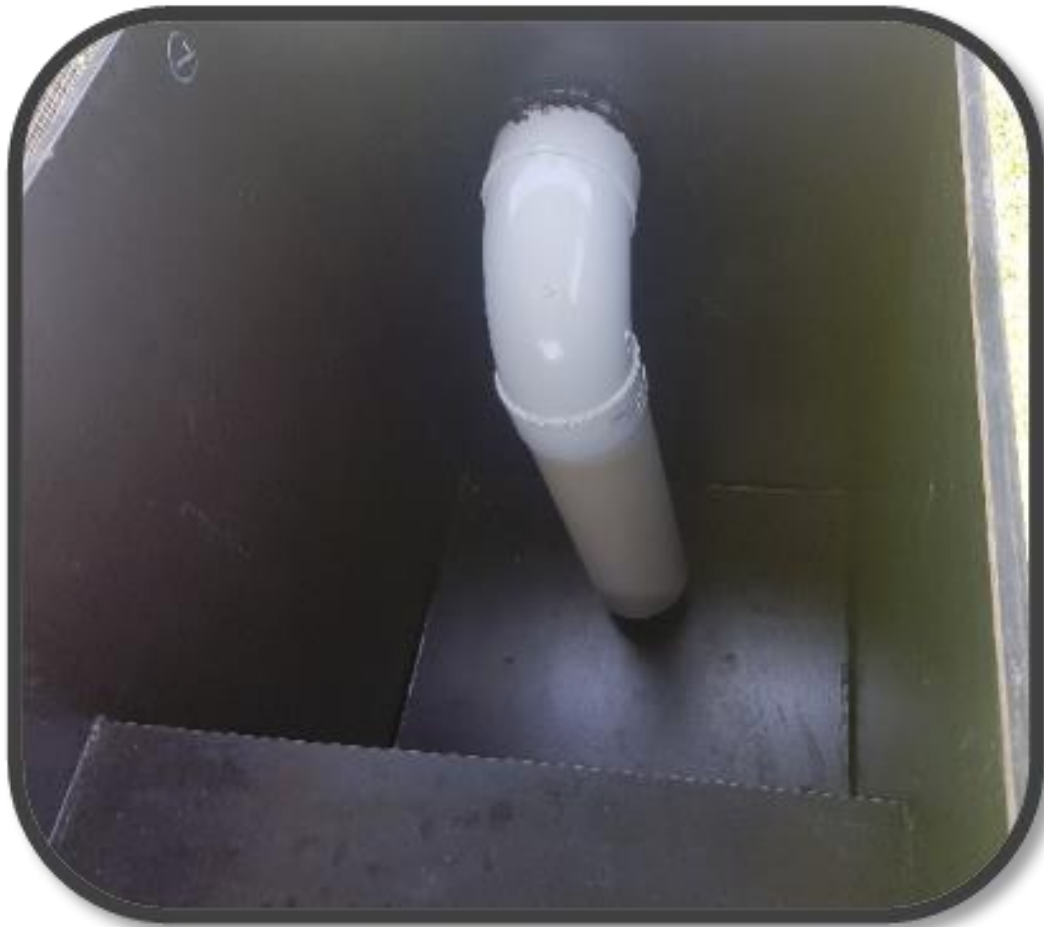
Figure 3.5: Containment flame trap (A Brian 2021, personal photograph, 22 September)
