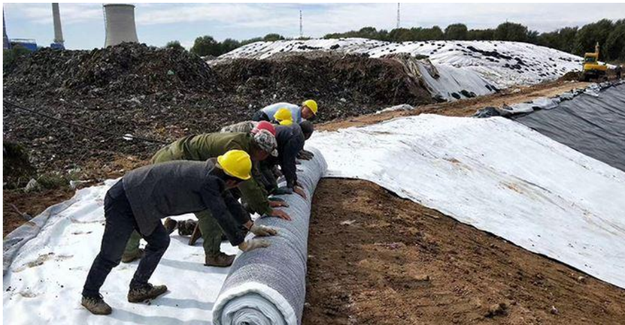
Figure 11. Installation of GCL in China. (MTTVS, 2021)
