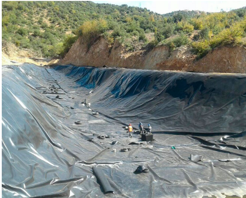
Figure 12. Installation of HDPE liners (Copin, 2019)
