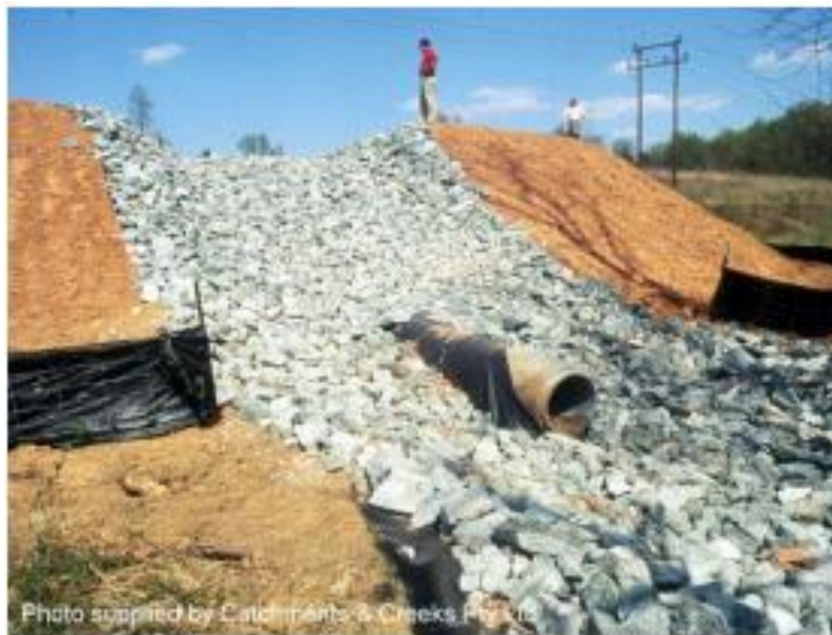
Figure 20. Example of spillway design. (Catchments and creeks, 2011)
